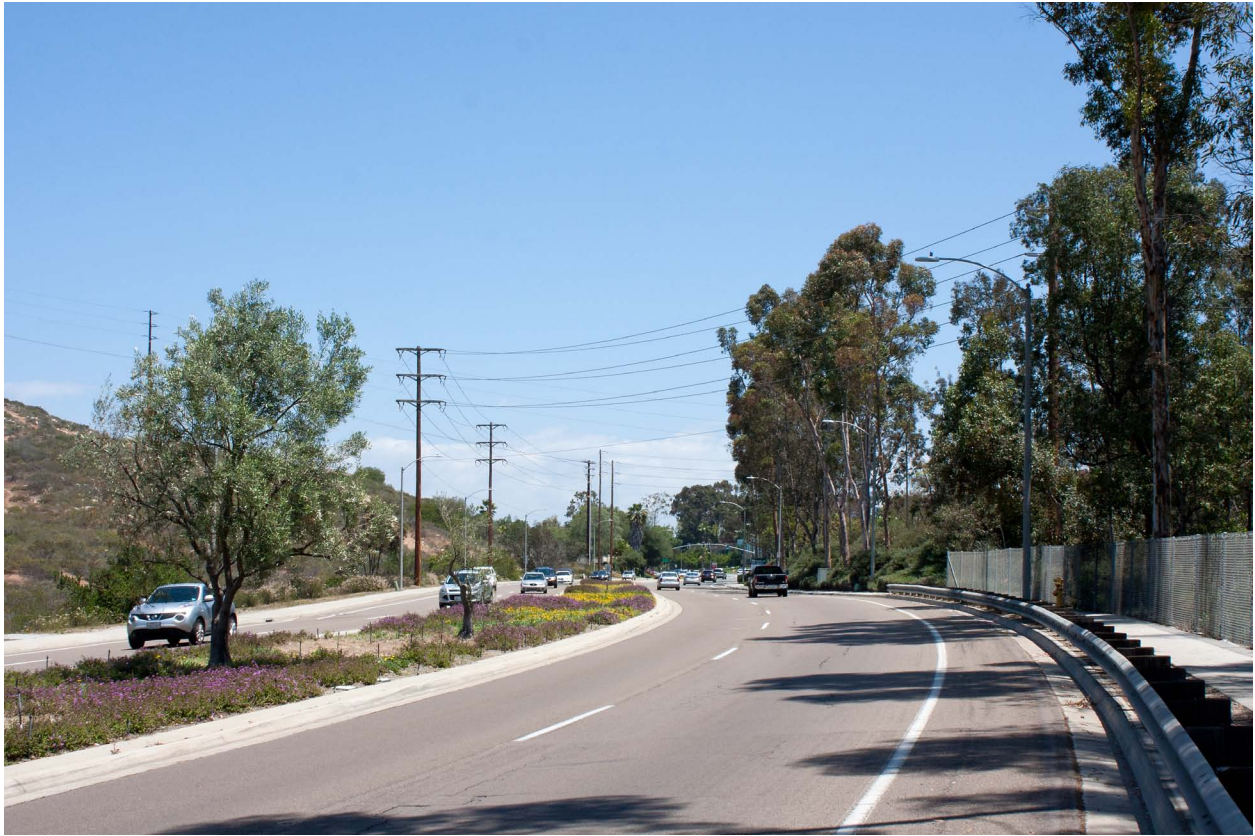
17. Rancho Bernardo Road near Camino San Bernardo looking northeast *
