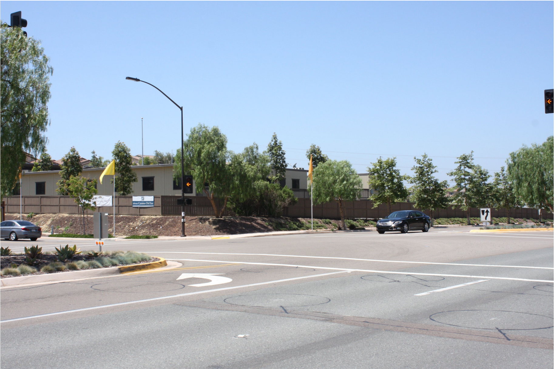
Existing view from Camino del Sur at Babcock Street looking southwest (VP 2)
