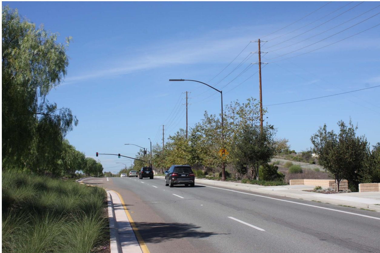
4. Camino del Sur near Babcock Street looking northwest *
