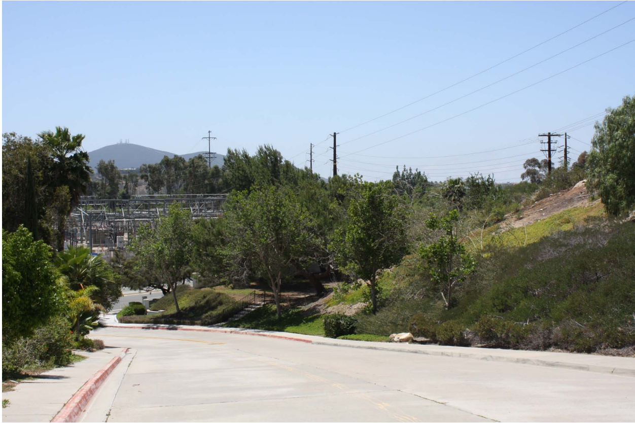
19. Via del Campo looking south towards Rancho Bernardo Substation
