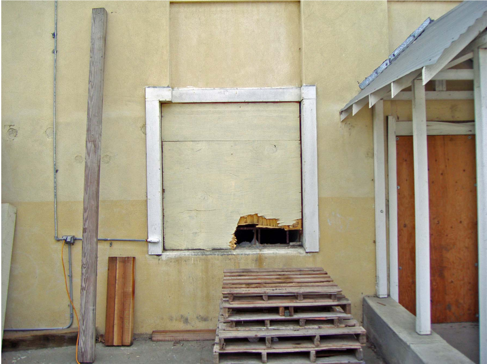
Altered Window on North Elevation of EII (facing South).
