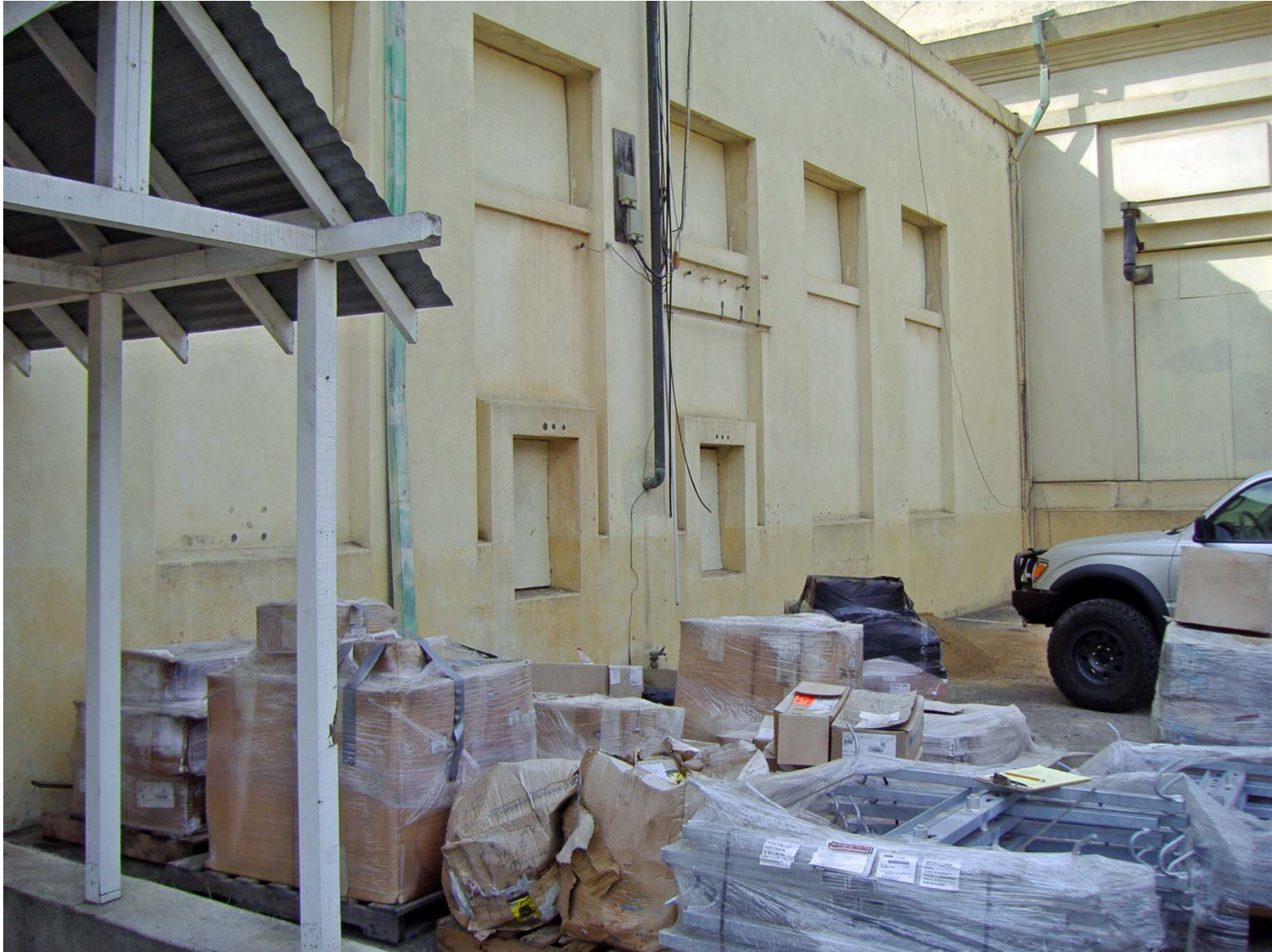
Overview of North elevation of EII, SD G & E (facing West/Southwest).
