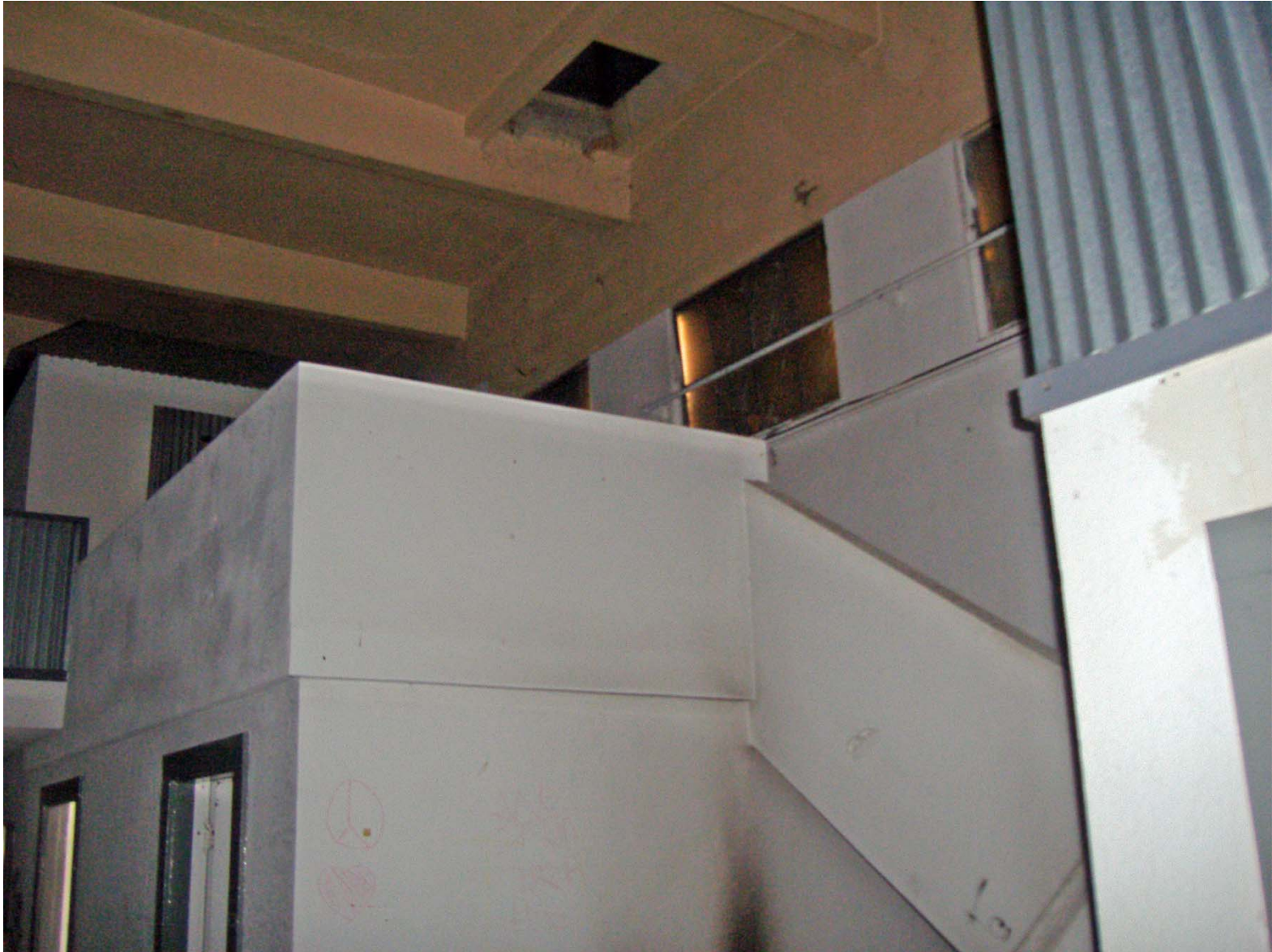
Stairway Leading to Second Story Offices (facing Northwest).
