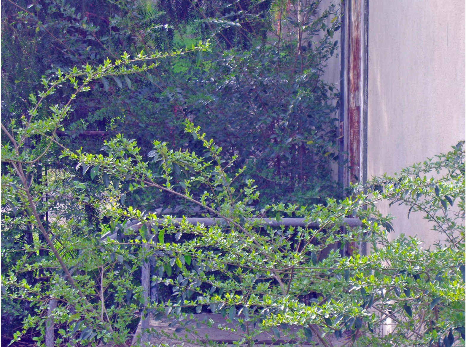
Exterior Door on East Elevation with Stoop and Railings (facing South).
