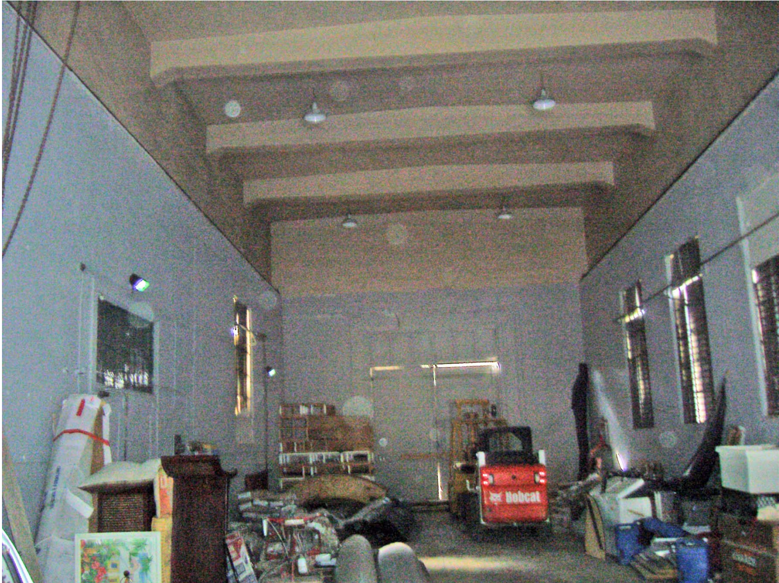
Interior of Main San Diego Gas & Electric Building, San Juan Capistrano (facing South).
