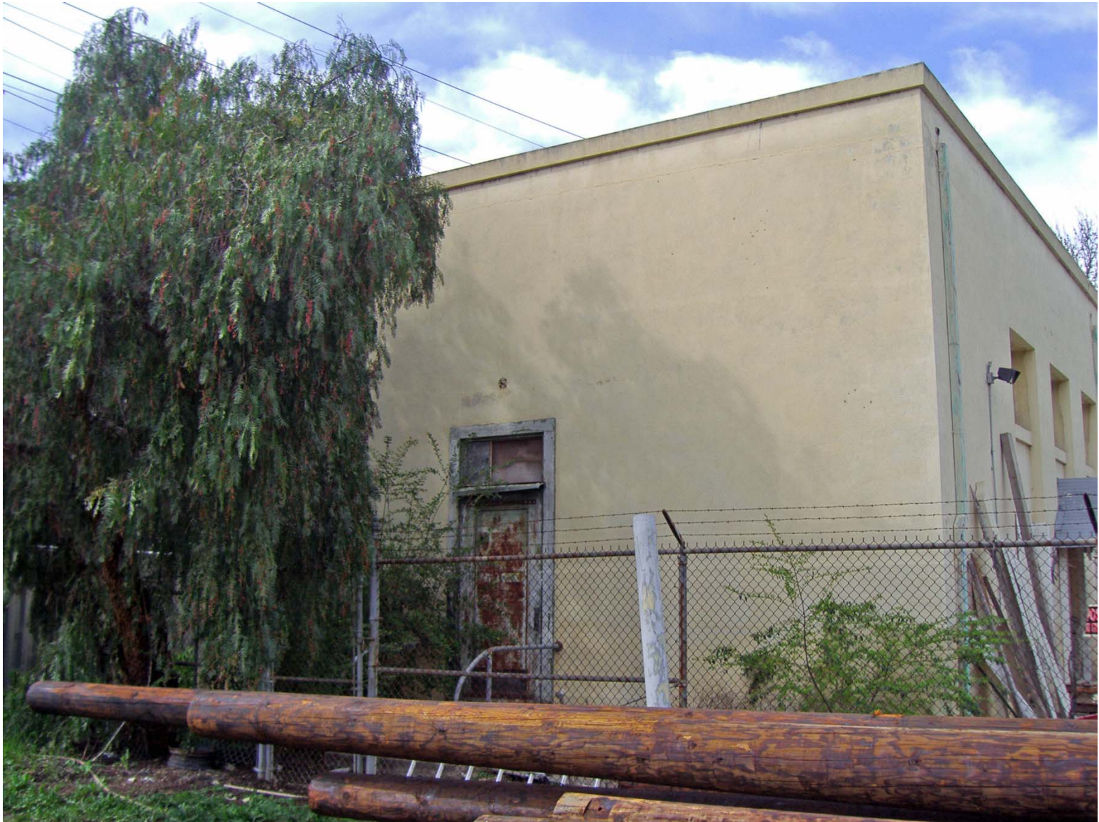
Overview of East Elevation (facing Southwest).
