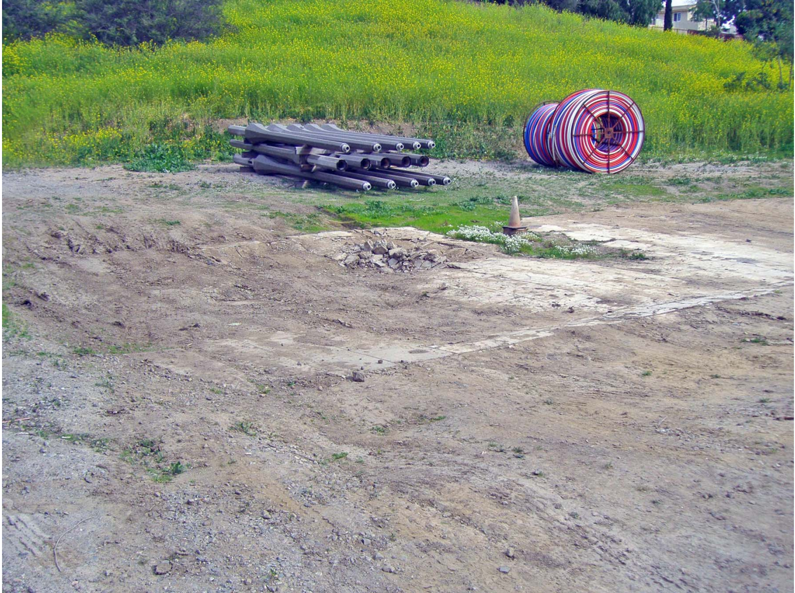
Broken Concrete Pad Identified as a Garage Area (facing Northeast).
