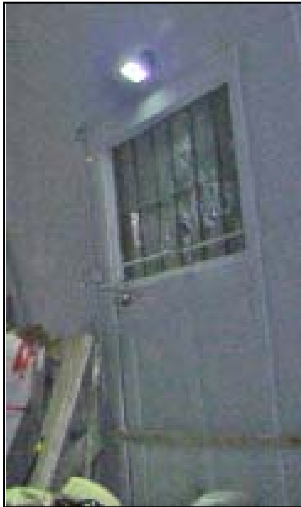
Figure 10. Interior Door on East Elevation.
