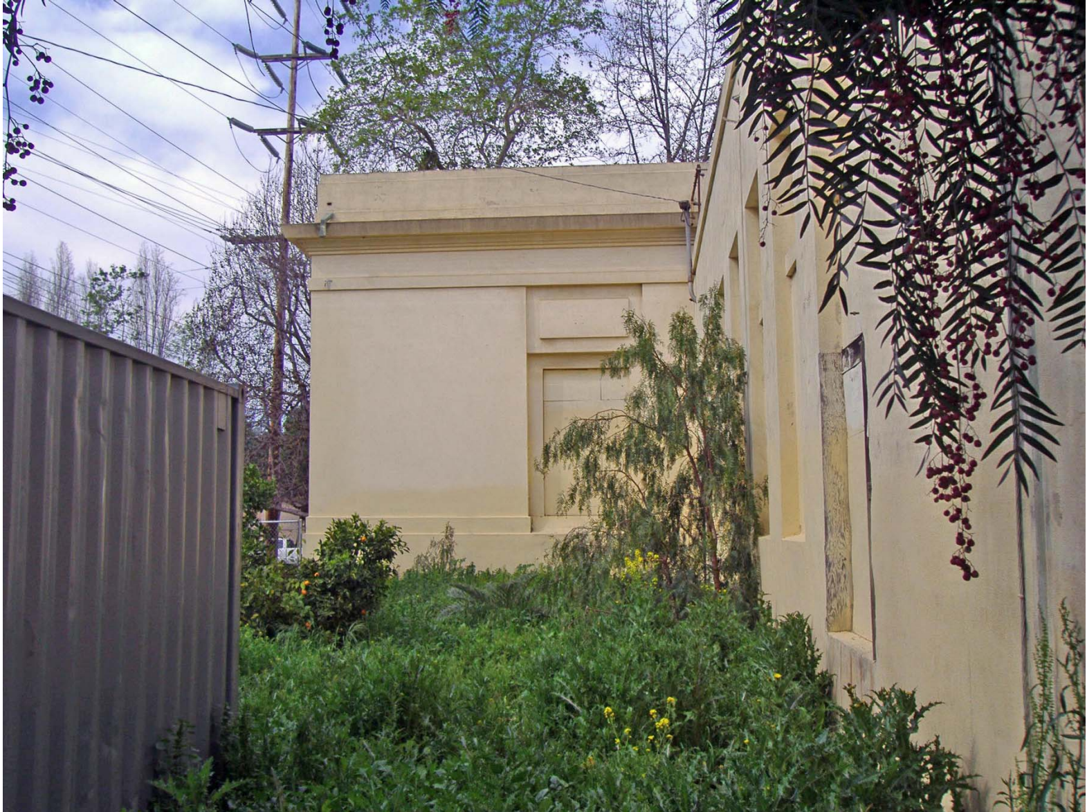
Overviedw of East Elevation of Main Building from East (facing West).
