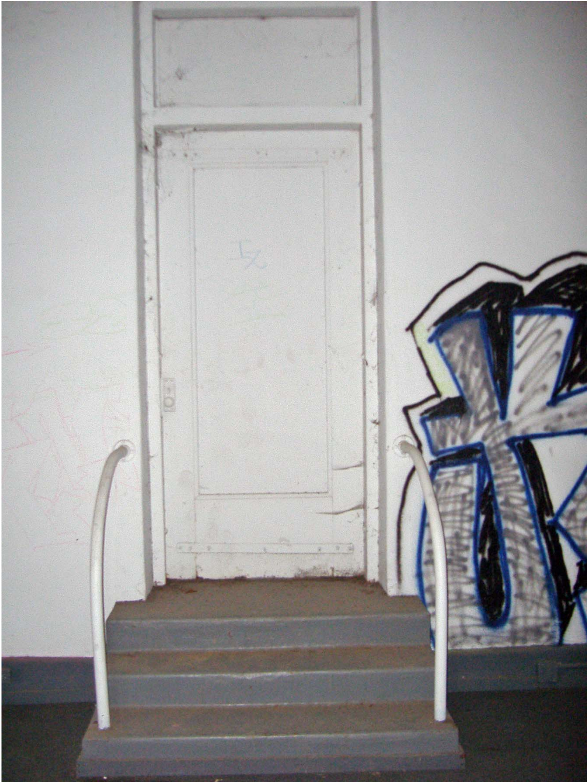
Exit Door on East Elevation of East Ell, SD G & E Building (facing East).
