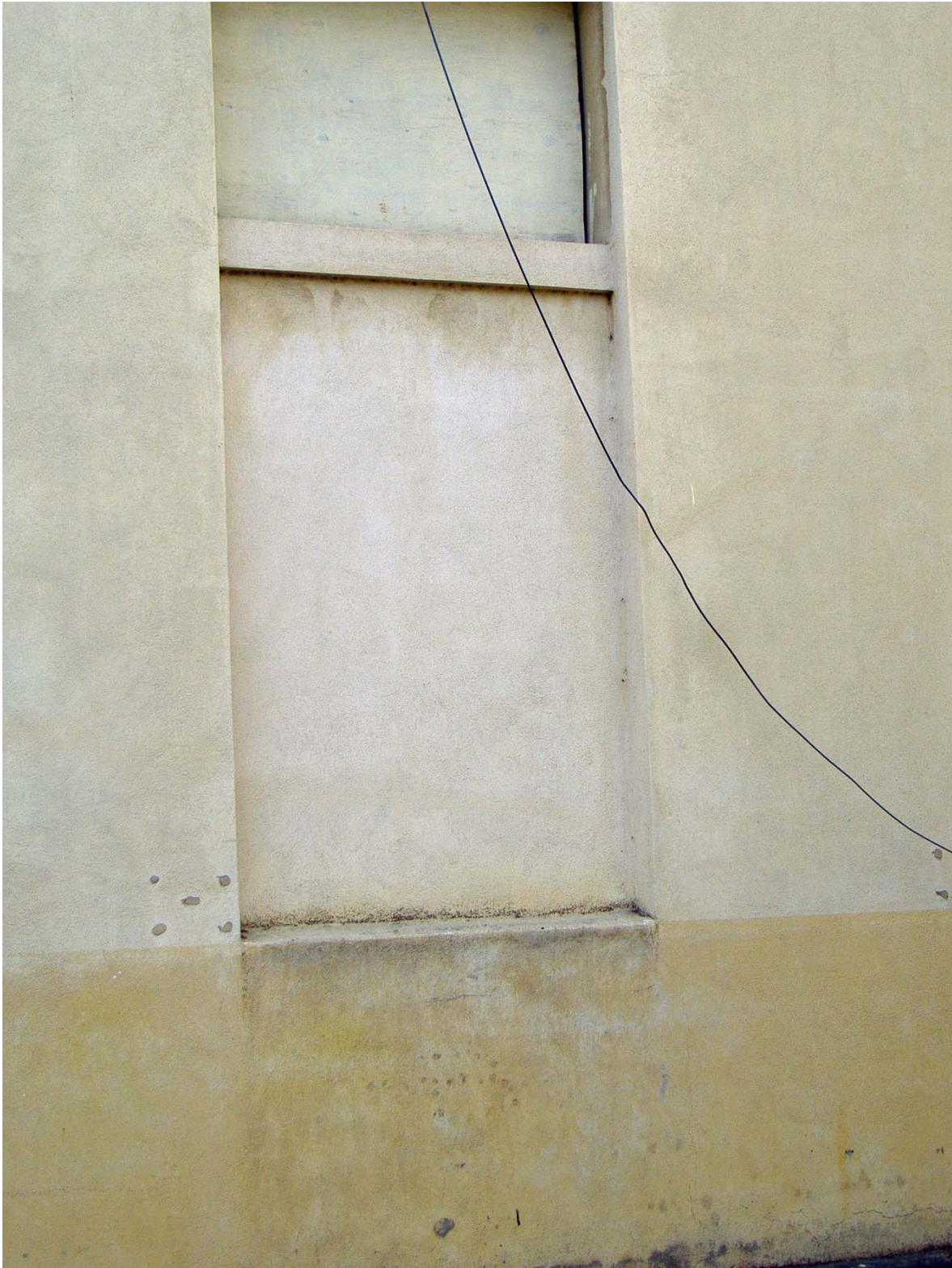
Example of Covered Window on North Elevation of E11 (facing South/Southwest).
