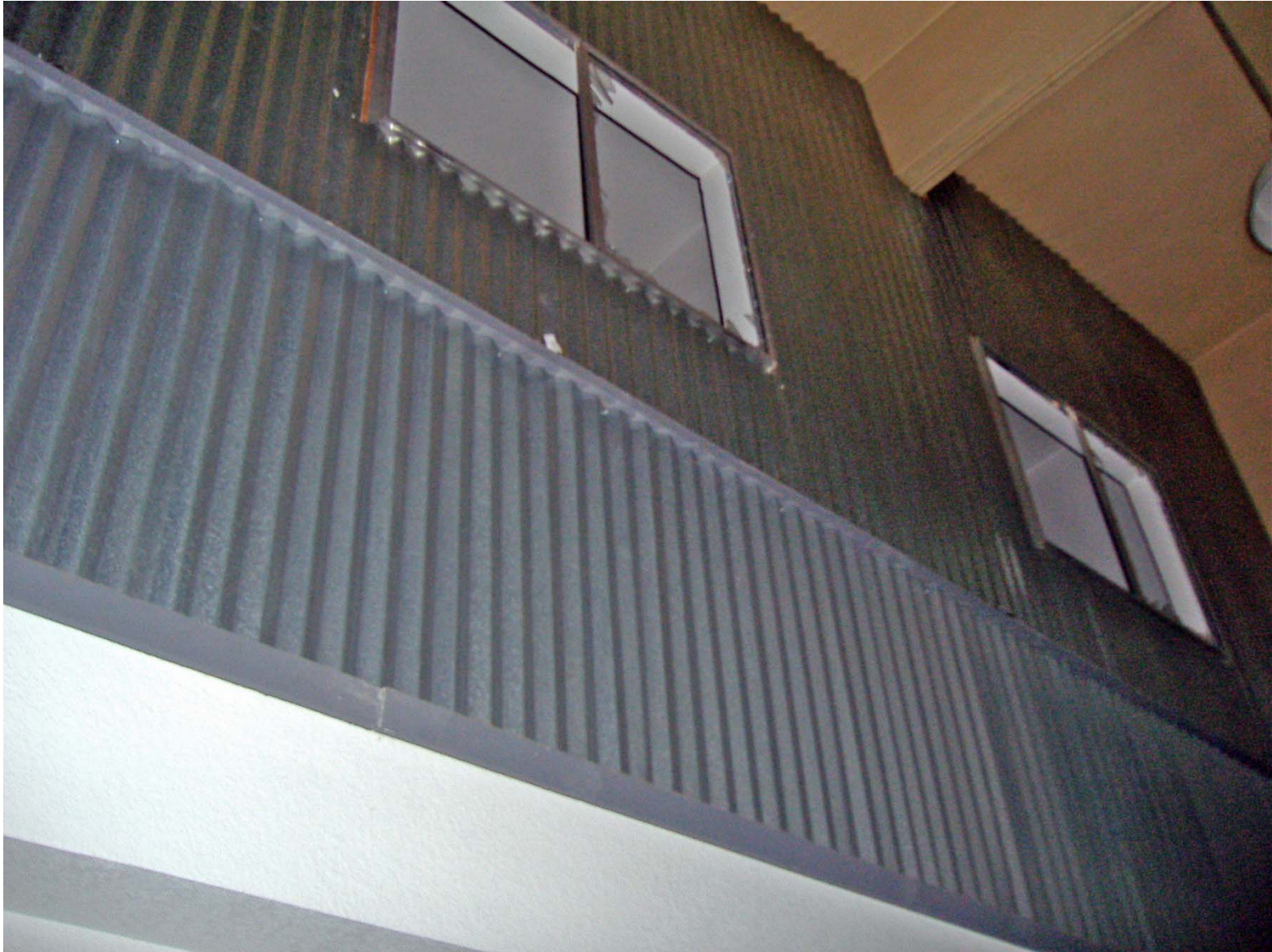
Second Story Offices (within East Ell (Original to Design; facing Southwest).
