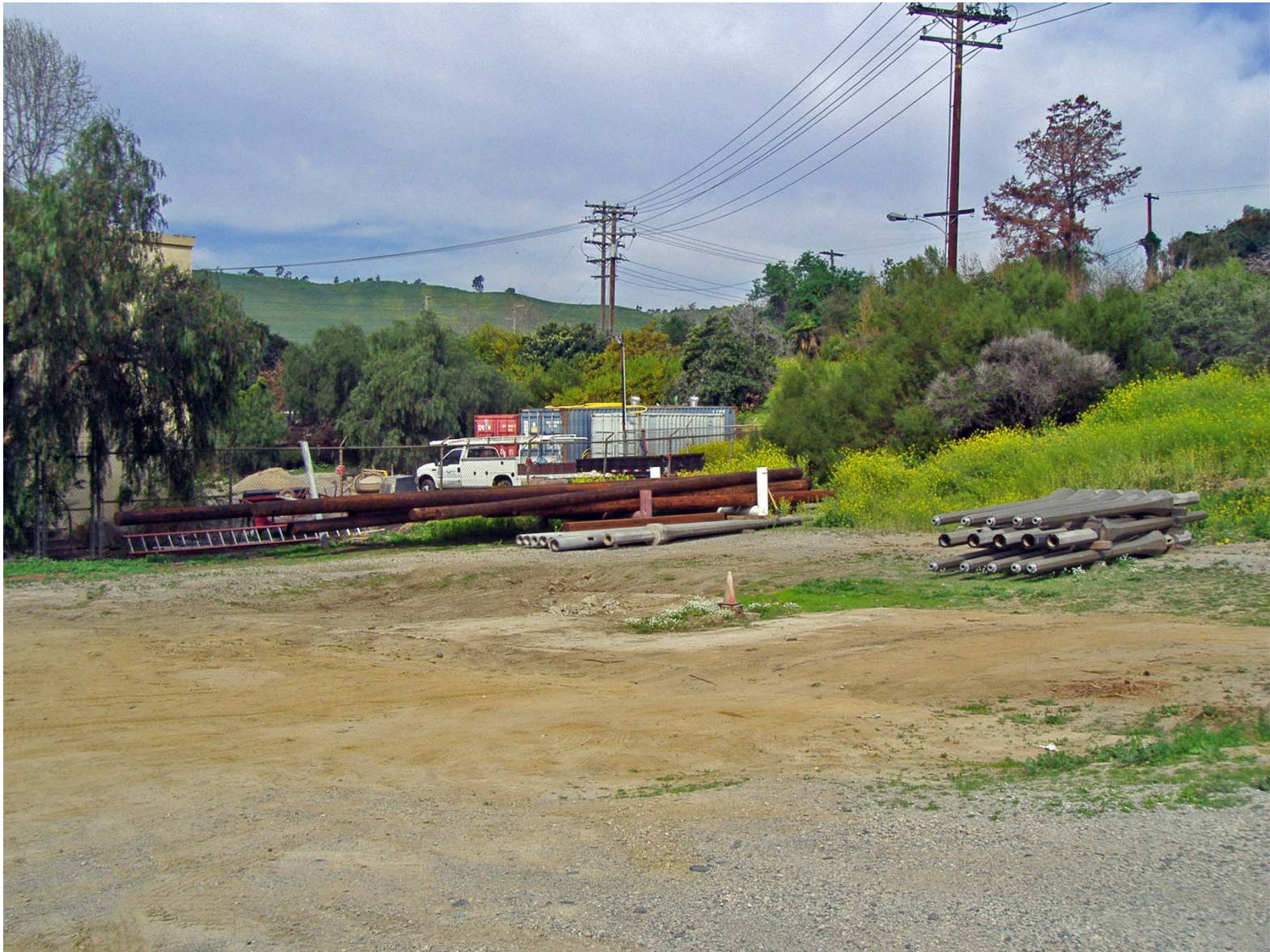
Overview of Yard Area Located North of the SD G & E Building (facing West/Northwest).
