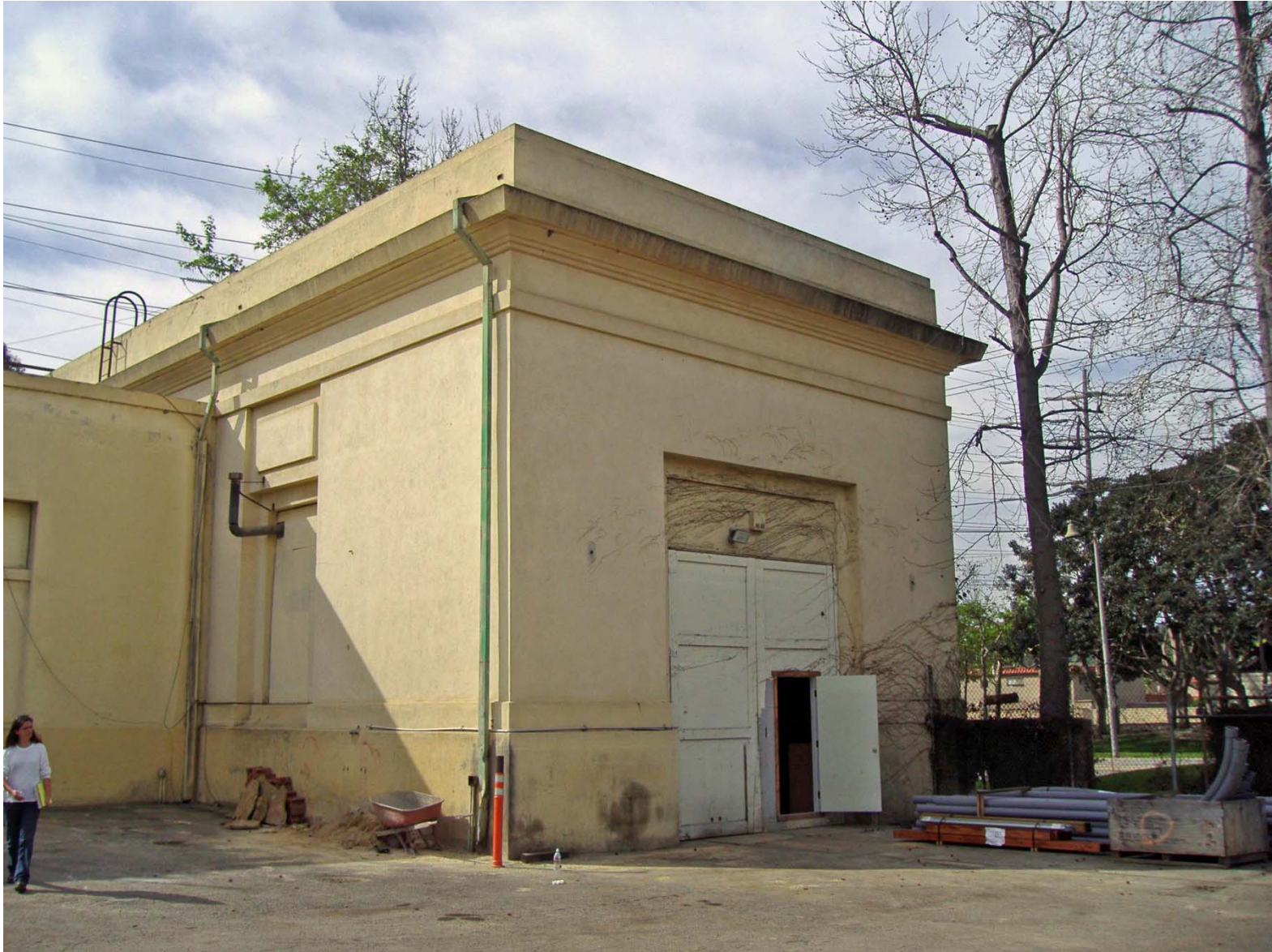
Overview of Eastern Extent of North Elevation of SD G & E Building, San Juan Capistrano (facing Northwest).
