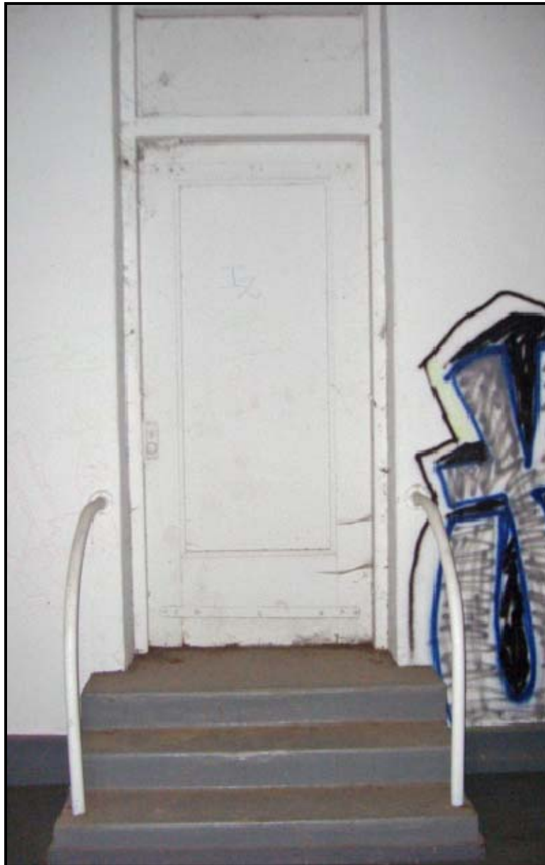
Figure 13. East Elevation Doorway from Interior of Building.
