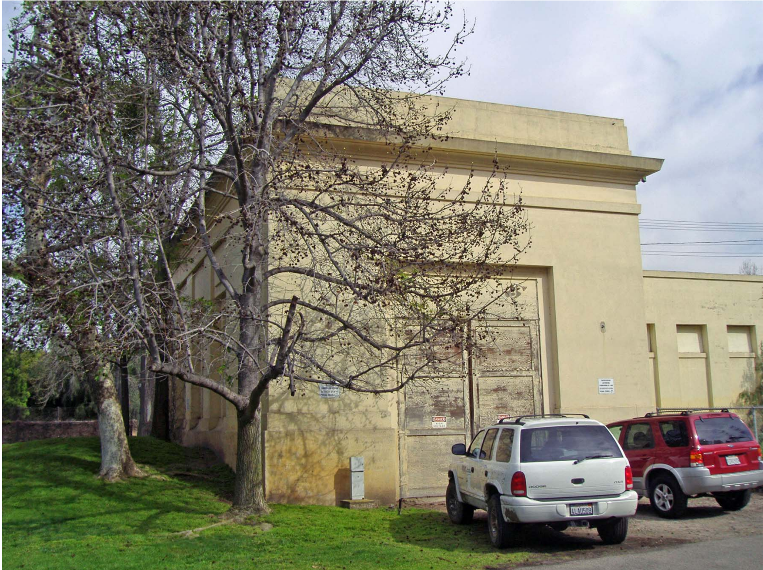
Overview of South Elevation of SD G & E Building (facing North/Northeast).
