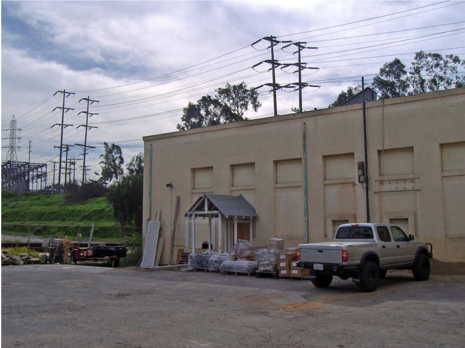
Overview of North Elevation of East EII, SD G & E Building (facing Southeast).
