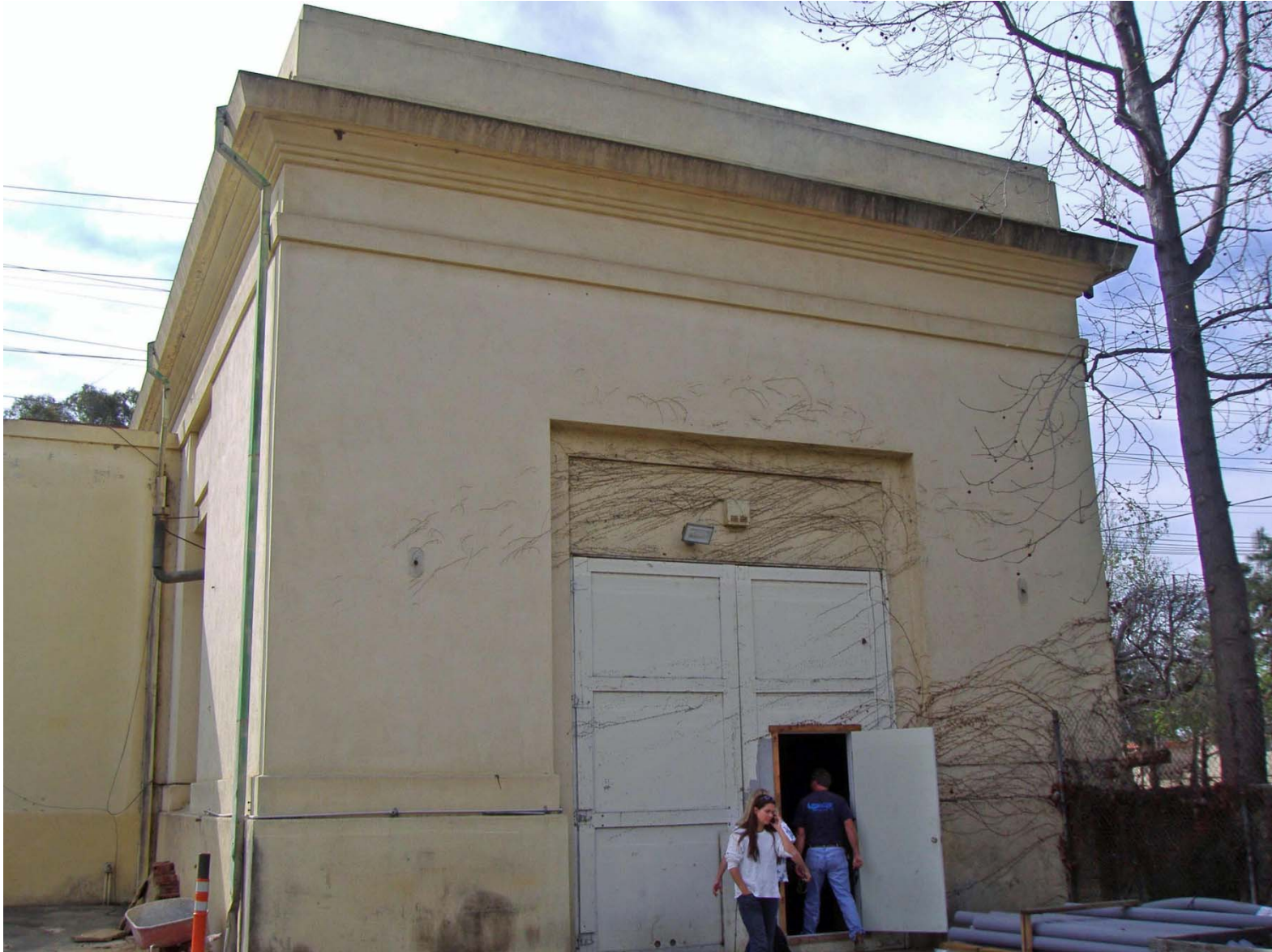
Detail of North Elevation (Small Door Added; facing South/Southwest).
