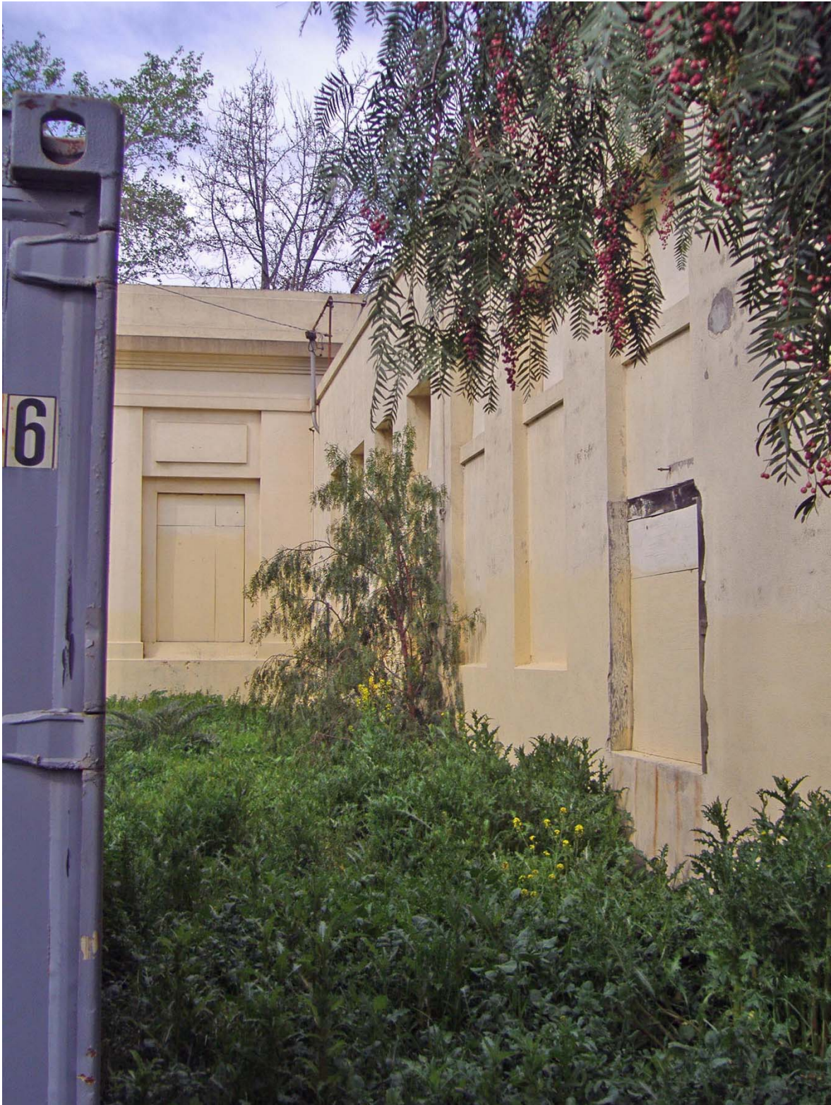
Overview of East El from South (facing North).
