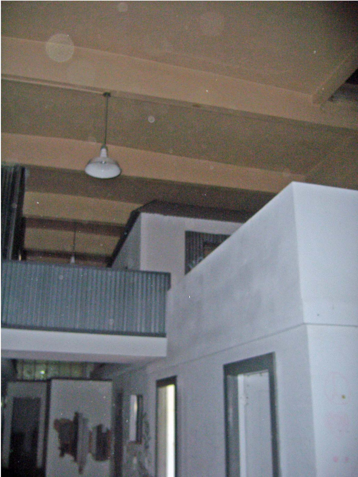
Overview of Second Story Offices (facing North/Northeast).
