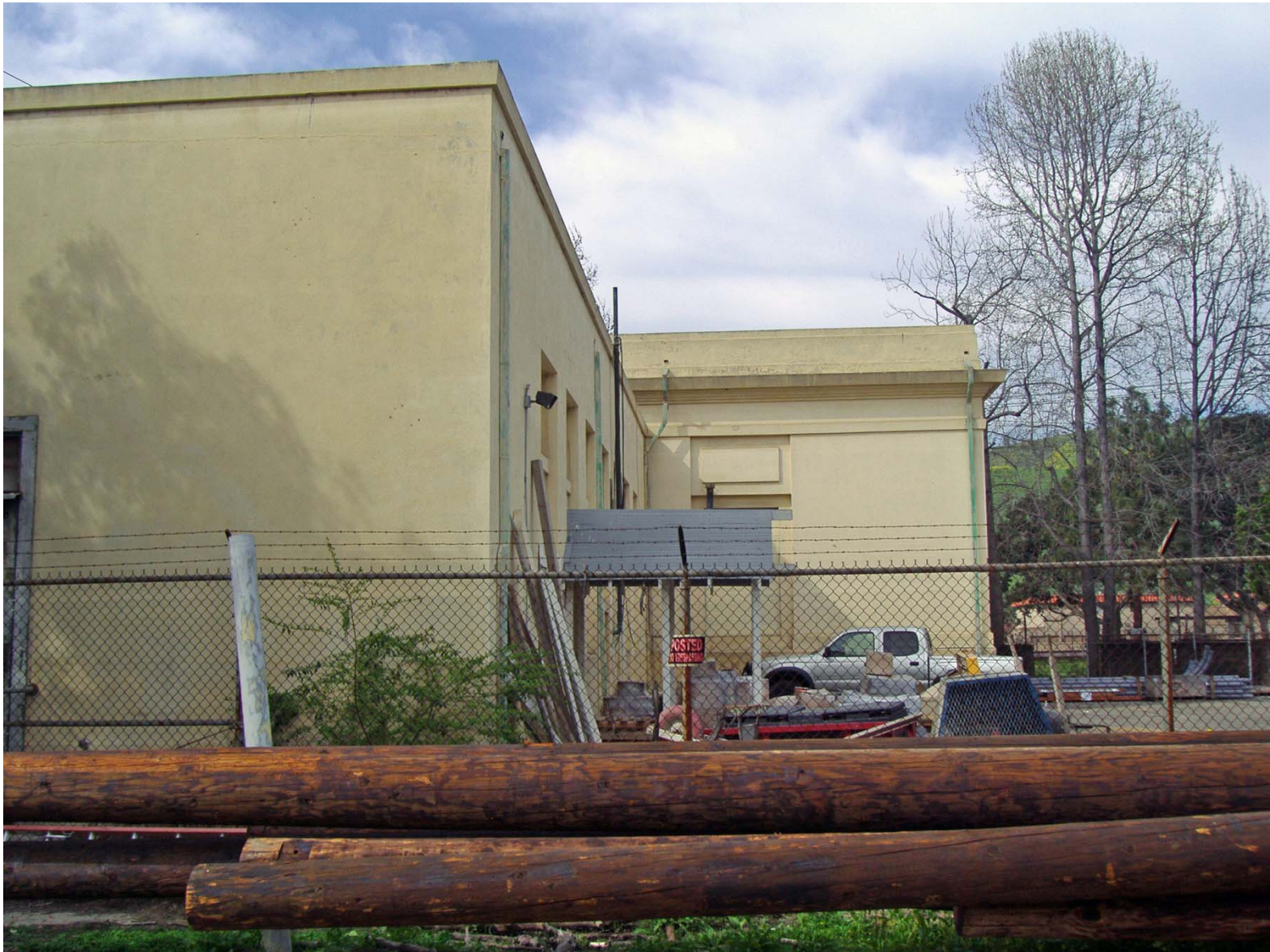
Overview of North and East Elevations from East (facing West).
