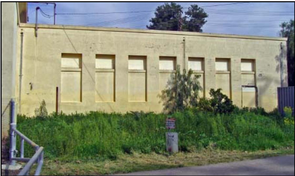
Figure 18. Overview of South Elevation of San Diego Gas & Electric Building.
