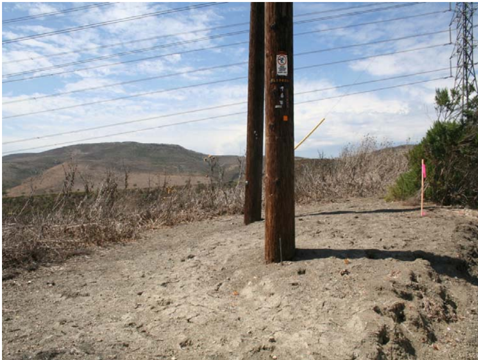
Photograph 2: Shows area of disturbance around pole location.
