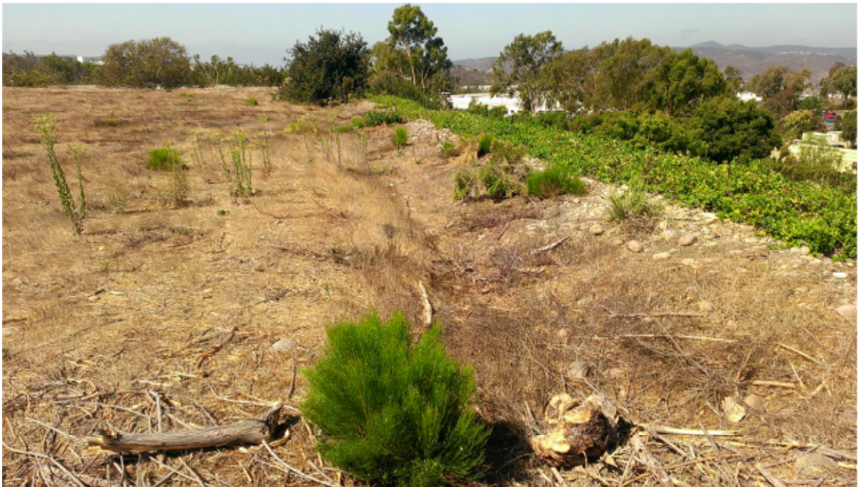
Photo 102: Stowe staging yard, erosion control ditch near the perimeter of the yard; Photo direction: NW
