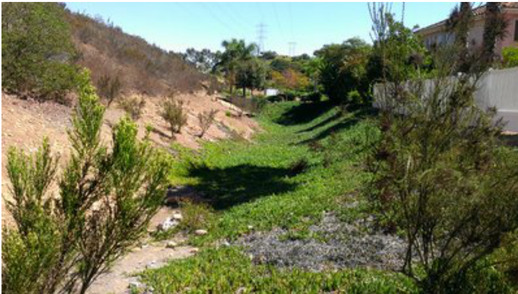
Photo 74: Cypress Canyon Feature 1, overview of iceplant-lined channel; Photo direction: NW
