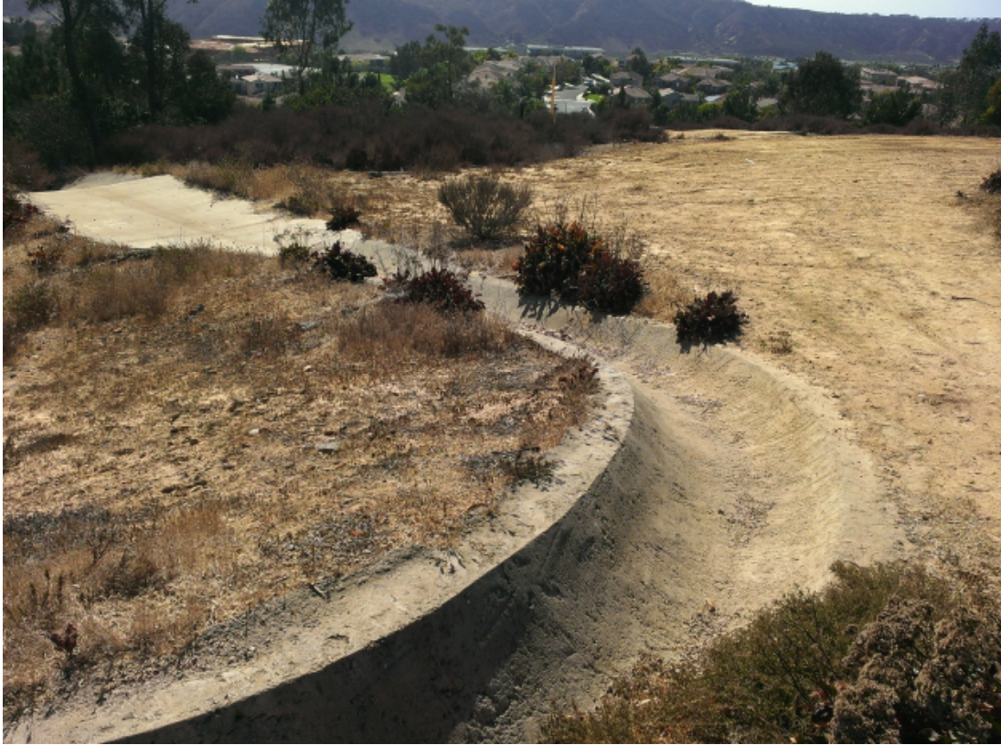
Photo 1: V-ditch draining the Peñasquitos substation pad; Photo direction: N
