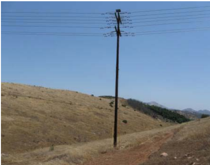
Illustration 2. Pole D28 facing north.
