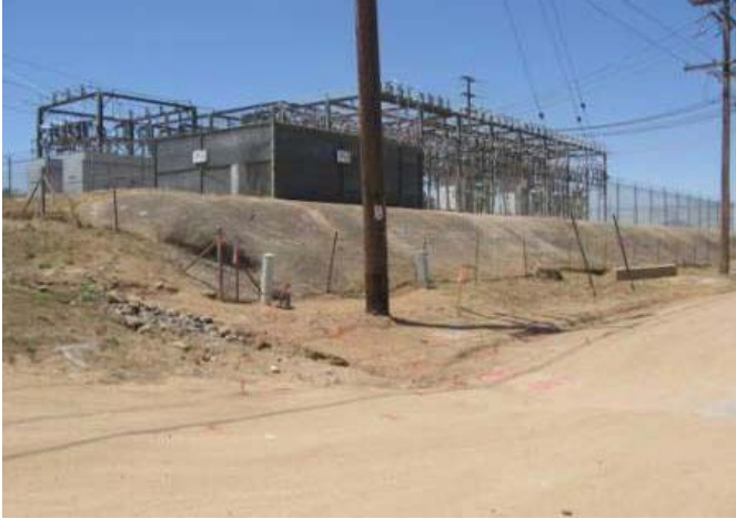
Illustration 1. Creelman Substation facing west.
