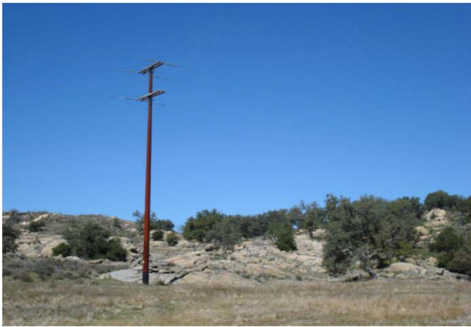
Illustration 14. View of TL 637 facing north.
