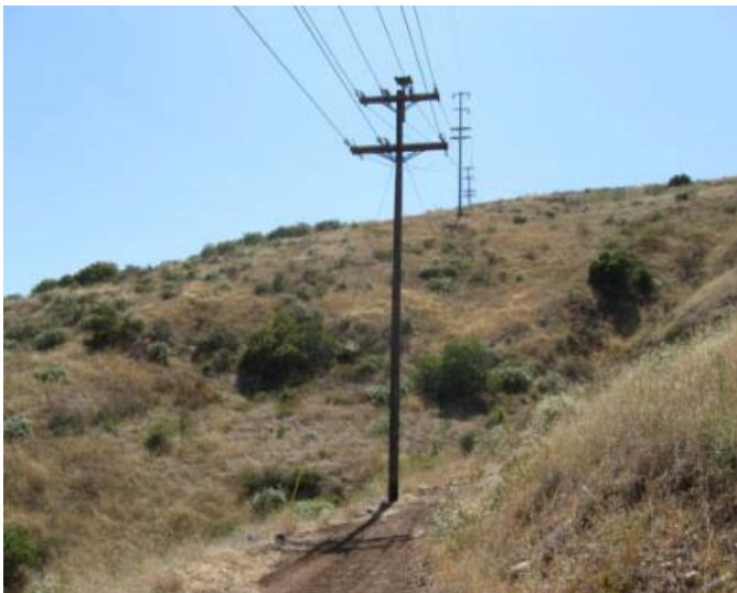
Illustration 3. Pole D31 facing northwest.
