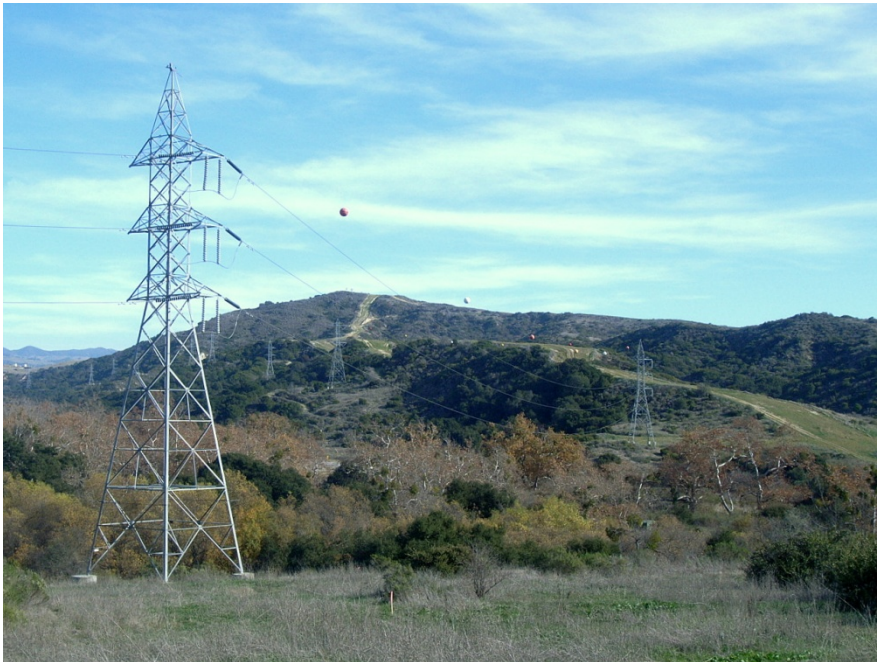
Photograph 6: View of riparian scrub south of the Talega substation. Riparian scrub
