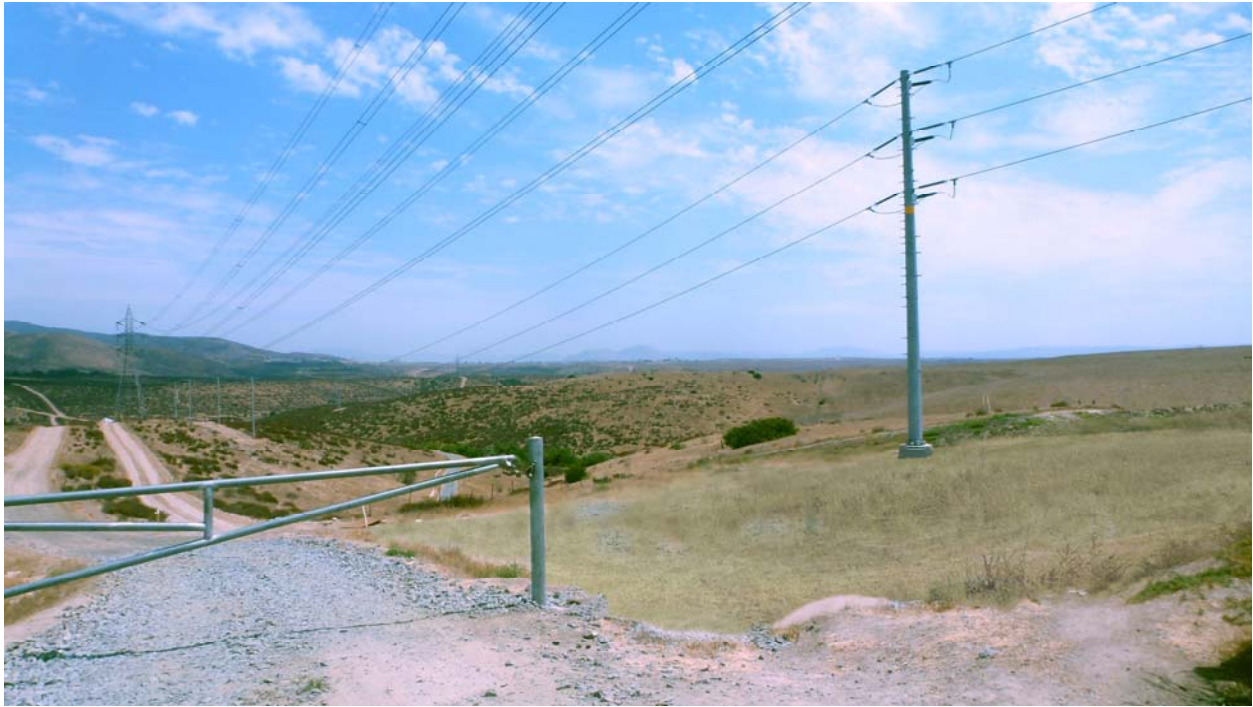
Figure 10: Key View 9: View Looking Southeast at Hunte Parkway/Transmission Corridor
