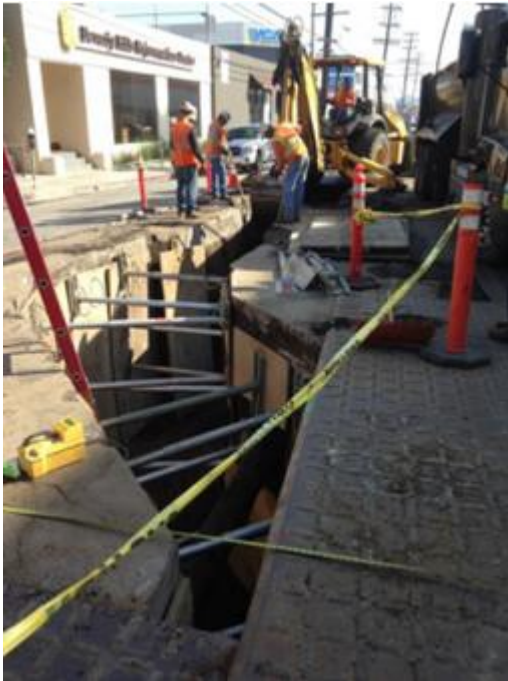
Figure 1: Trenching in Urban Location
