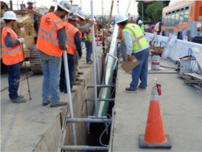
Figure 2: Lowering Pipe in Congested City Area
