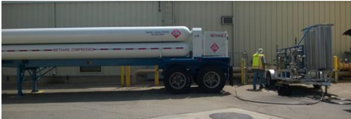
Figure 15: CNG for Temporary Bypass
