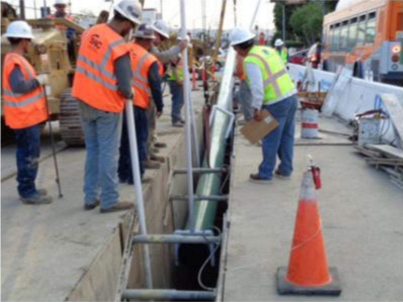
Figure 2: Lowering Pipe in Congested City Area
