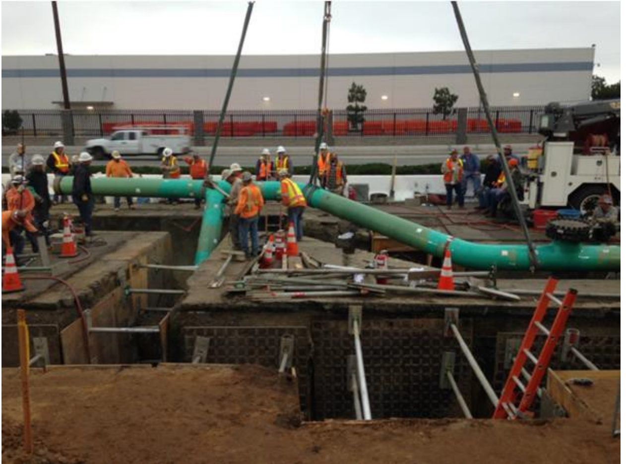
Figure 9: Lowering Section of Pipe into Trench
