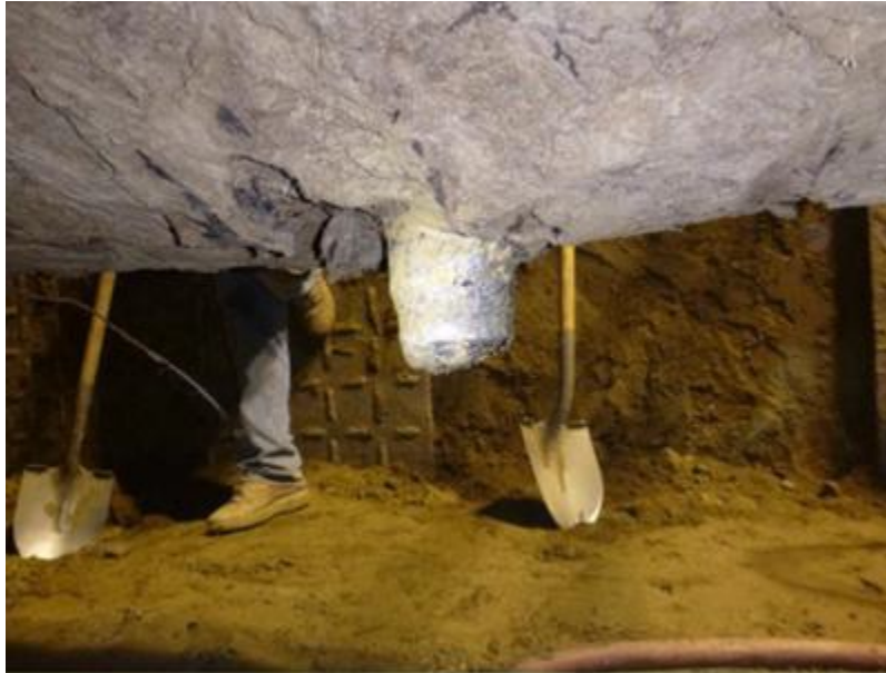
Figure 14: Feature to be Removed from L-2000W Before Hydrotest
