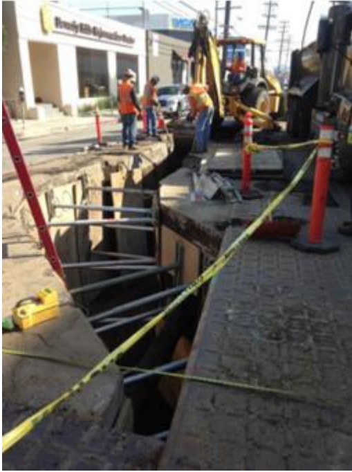
Figure 1: Trenching in Urban Location
