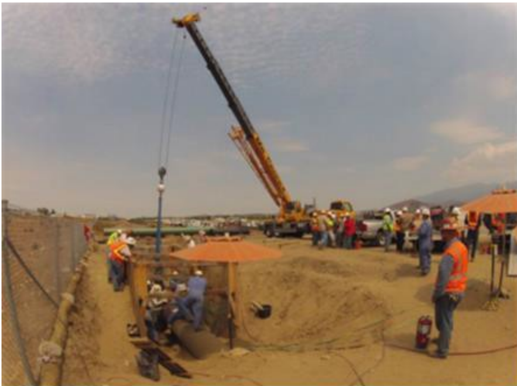
Figure 13: L-2000 Tie-In Construction
