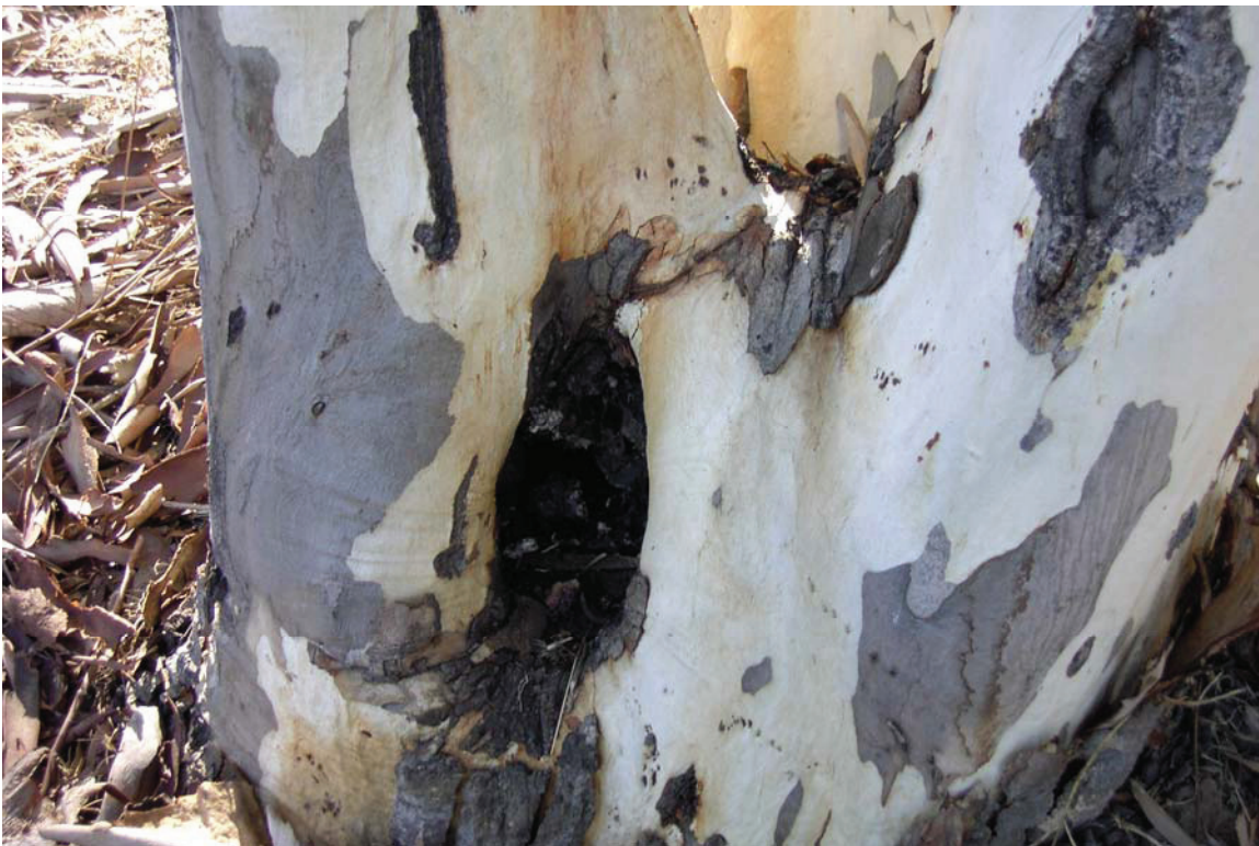
Figure 11: Interior rot at base of eucalyptus that may lead to future failure.
