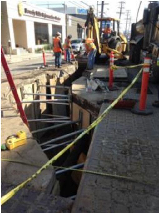
Figure 1: Trenching in Urban Location
