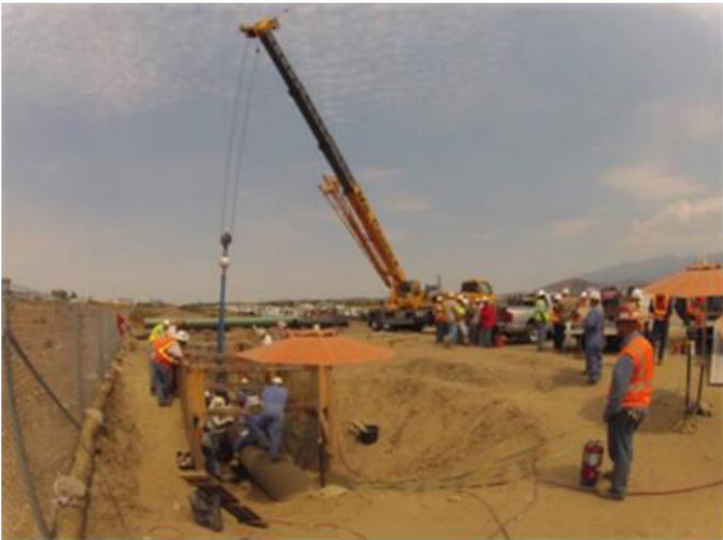
Figure 14: L-2000 Tie-In Construction
