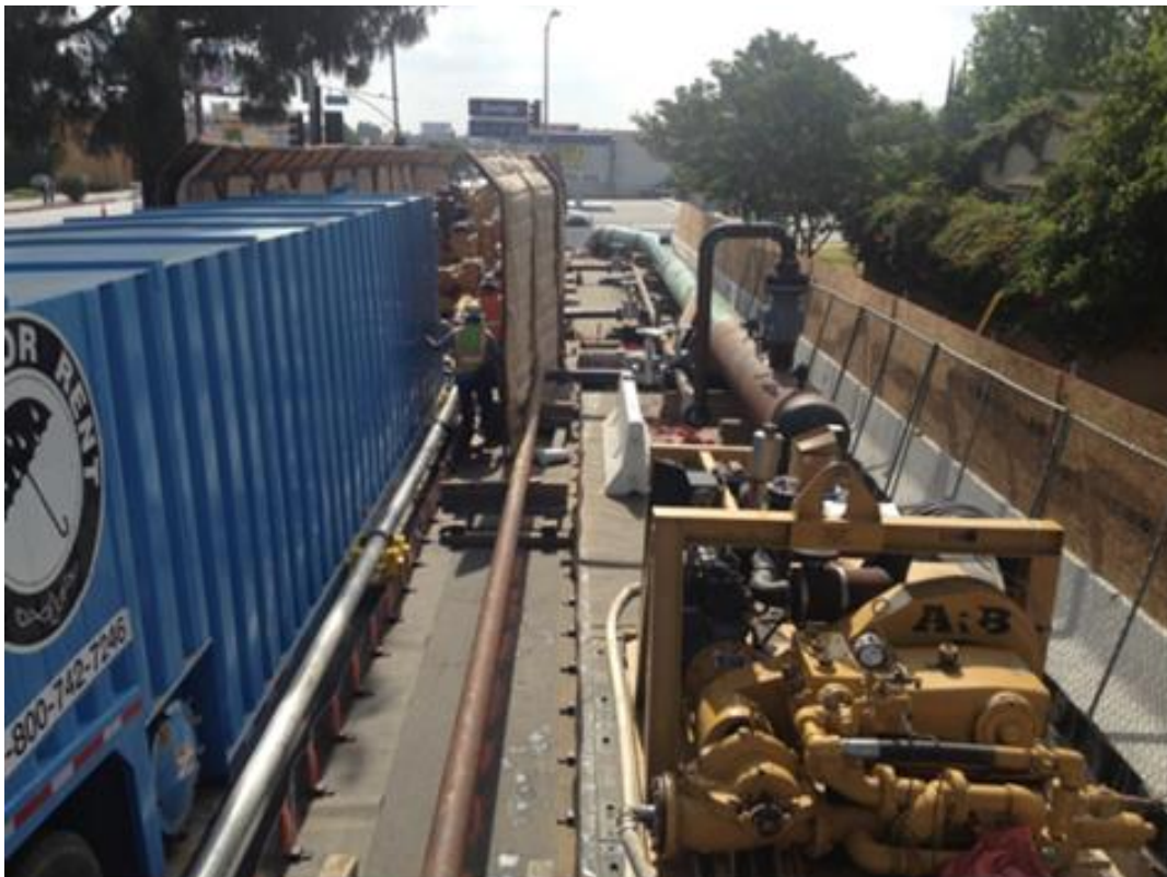
Figure 12: Hydrotest Set Up with Sound Proofing to Minimize Noise Complaints (located behind Baker tank)
