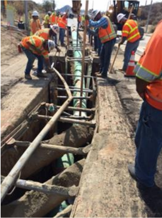
Figure 3: Installing Pipe in Trench with Existing Substructures
