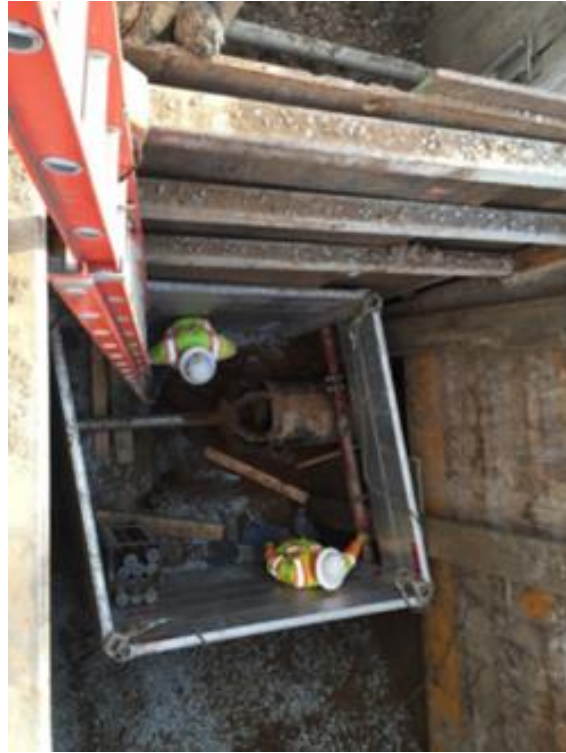
Figure 7: Jack and Bore Pit
