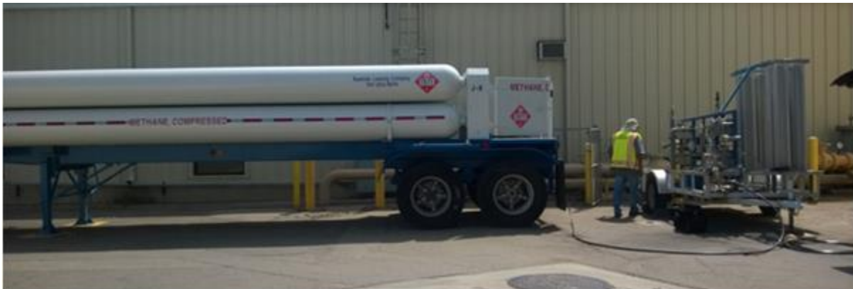
Figure 16: CNG for Temporary Bypass
