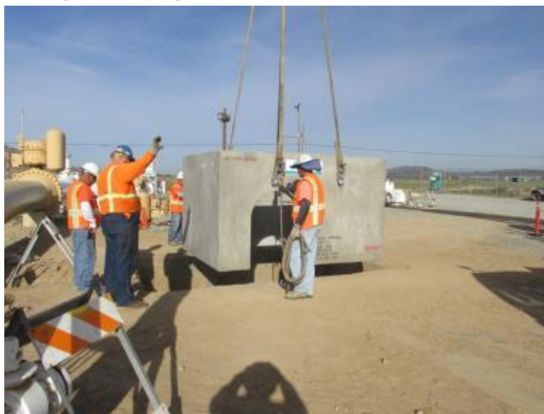
Figure 2: Image of Installation of Concrete Vault
