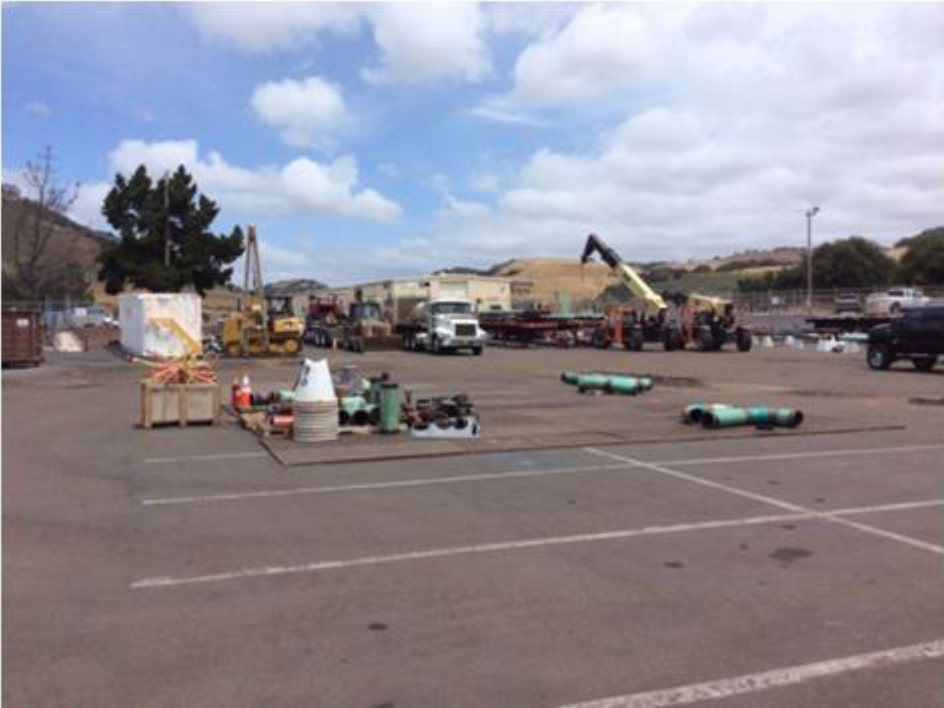
Figure 5: Construction Laydown Yard
