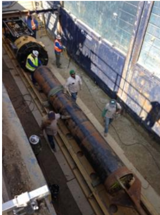
Figure 8: Jack and Bore Operation
