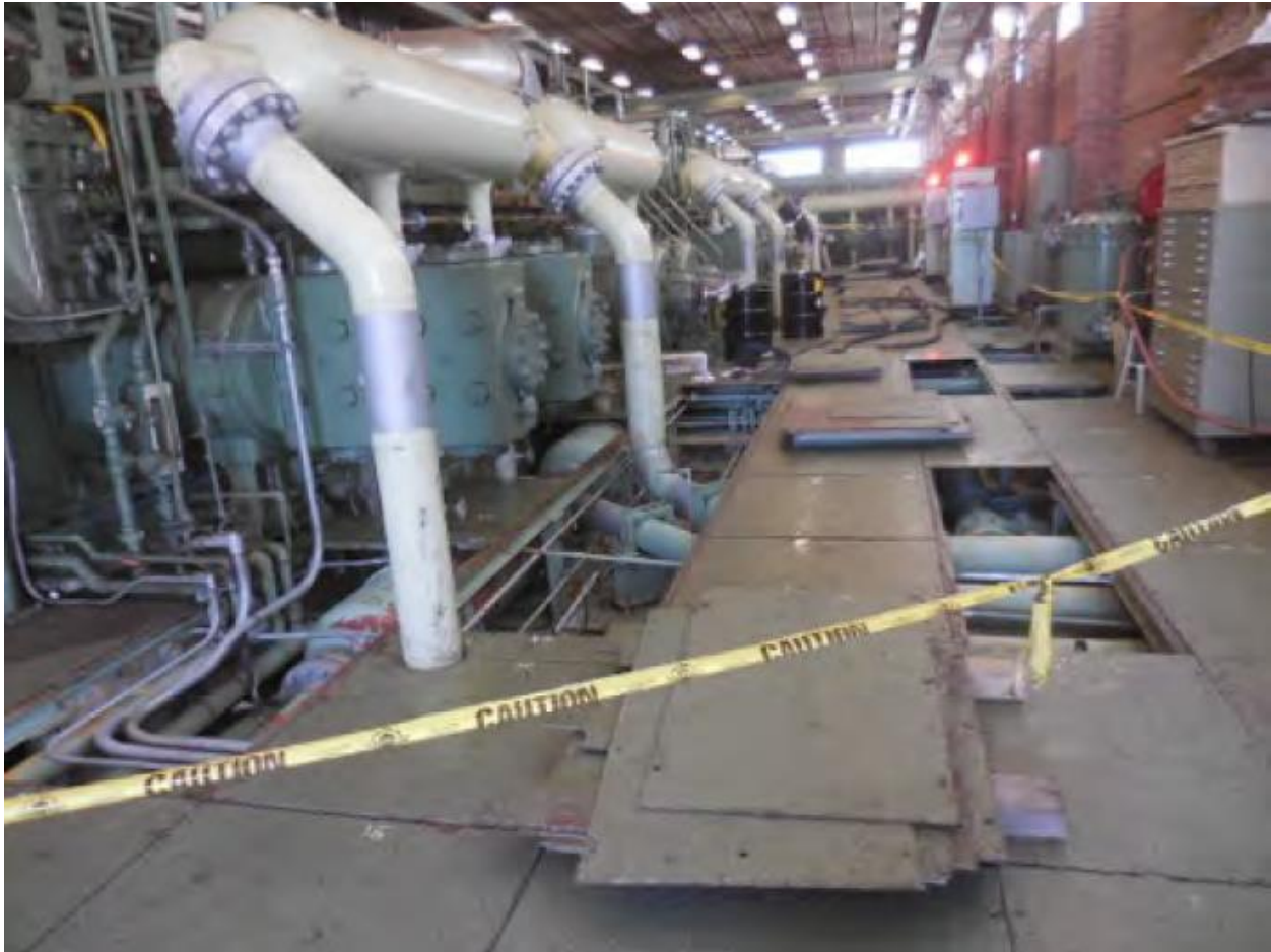
Figure 3: Exposing Compressor Injection Piping in Preparation for Test
