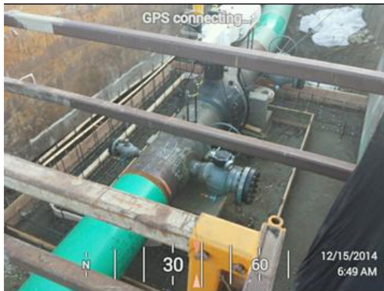
Figure 9: 2001 W Section 10 MLV Installation and Shoring for Vault Construction
