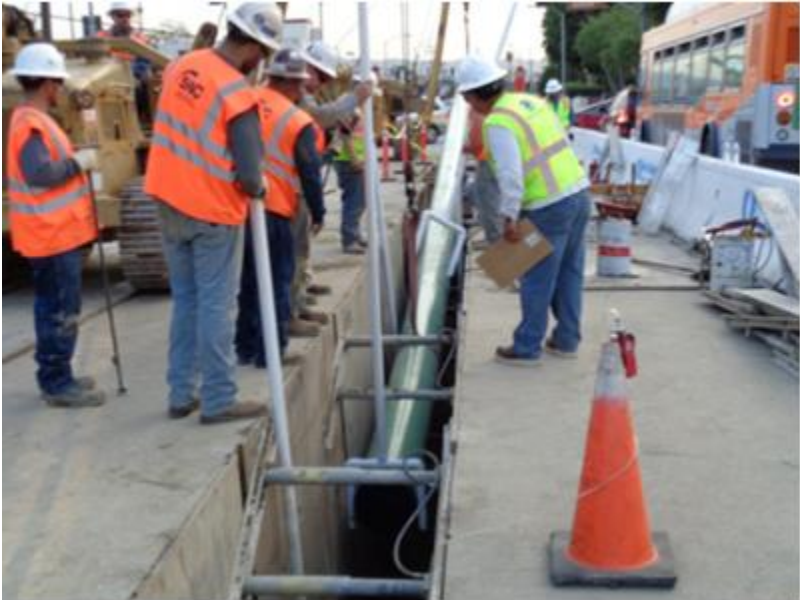
Figure2: Lowering Pipe in Congested City Area
