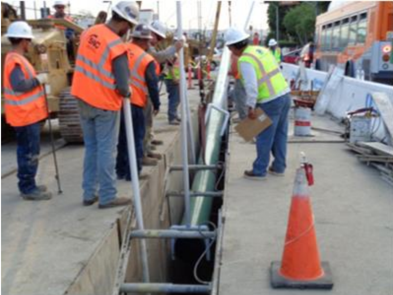
Figure2: Lowering Pipe in Congested City Area
