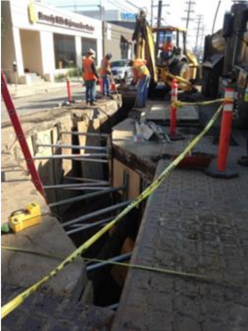
Figure 1: Trenching in Urban Location
