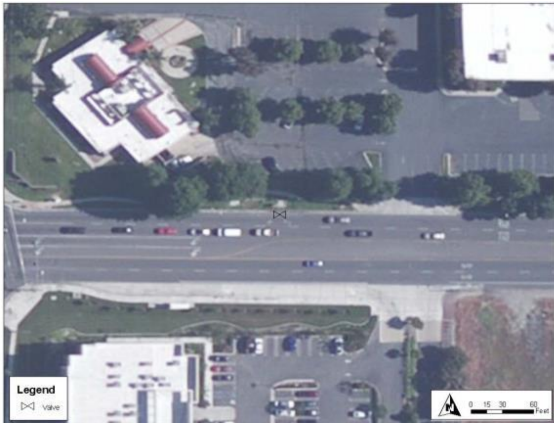
Figure 1: Satellite Image of Arrow & Haven Valve Project
