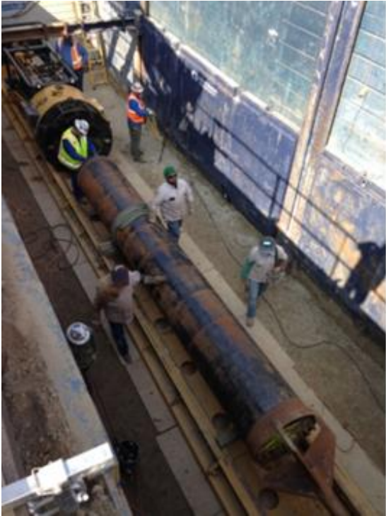
Figure 8: Jack and Bore Operation
