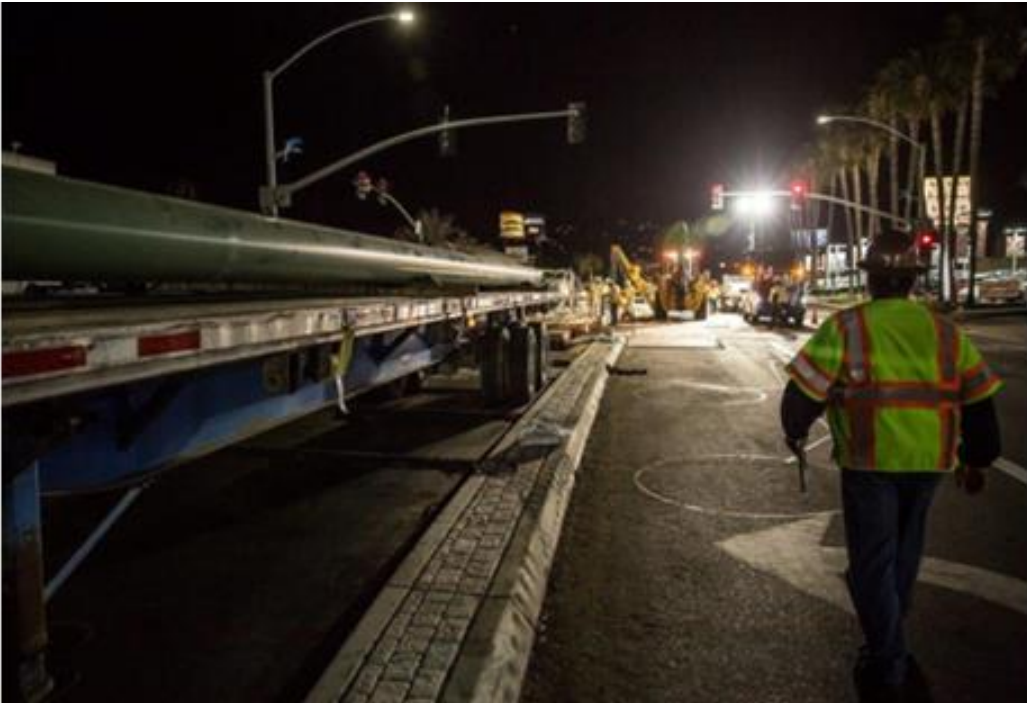
Figure 4: Night Work Construction Site
