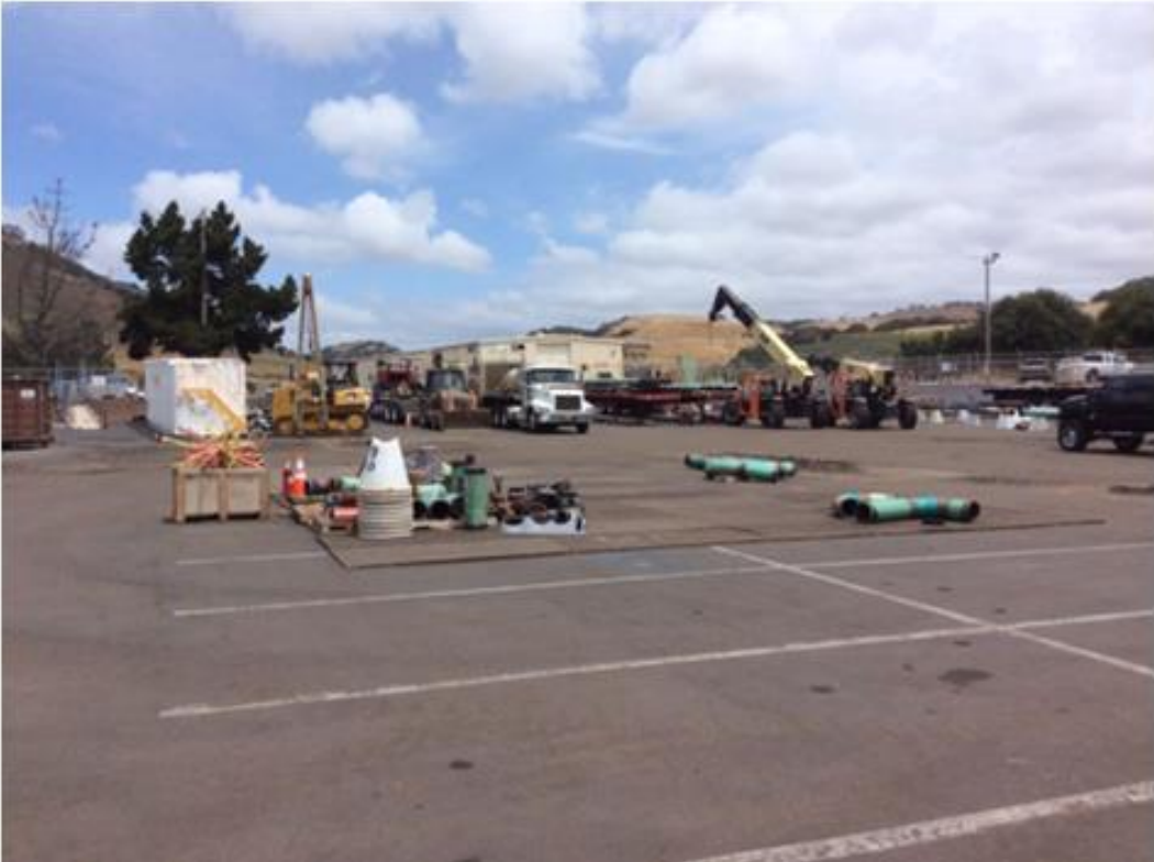
Figure 5: Construction Laydown Yard
