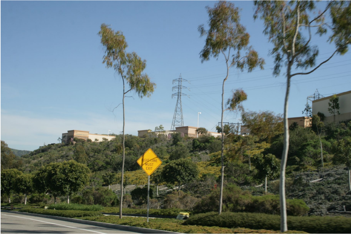
33. Avenida Pico near Camino Celosia looking southeast
