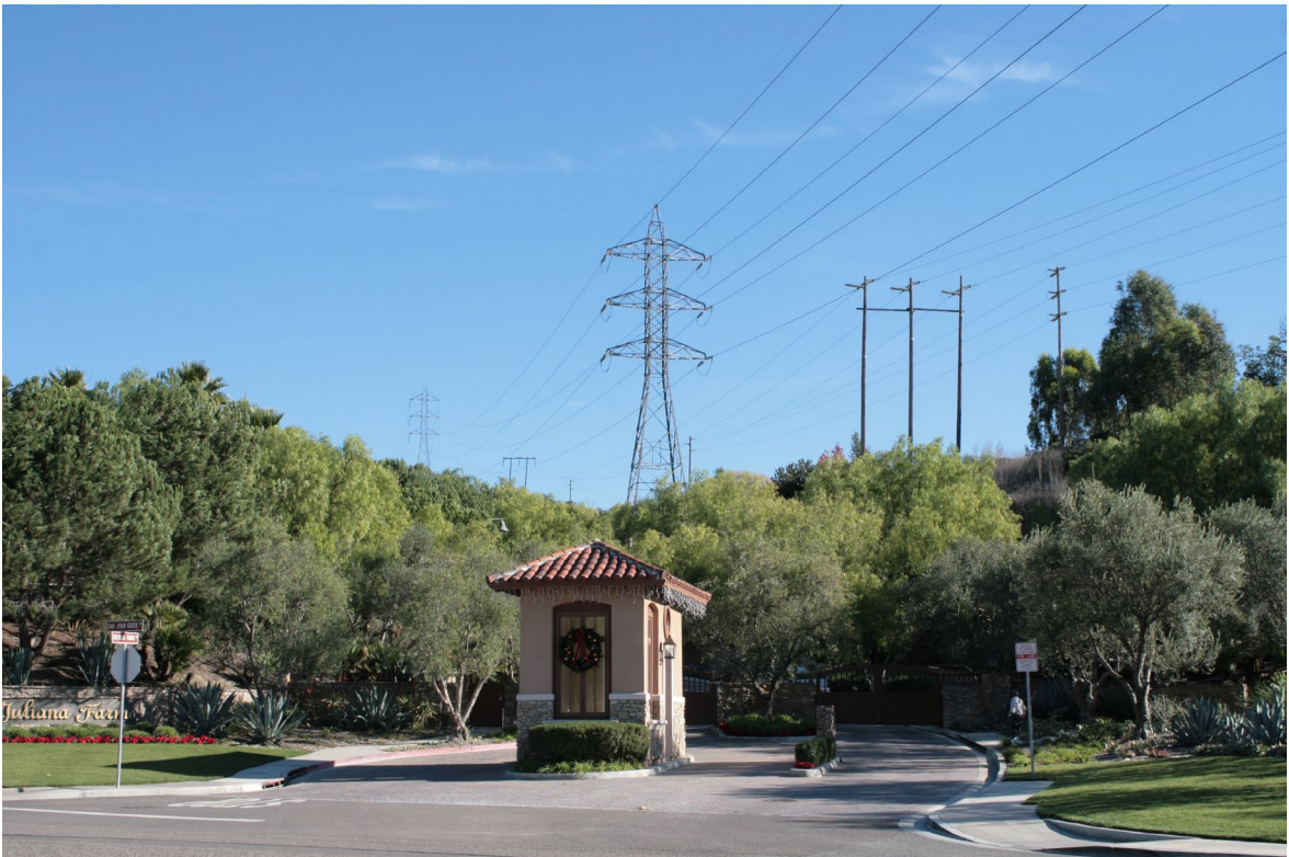
20. San Juan Creek Road at Juliana Farms Road looking southeast*
