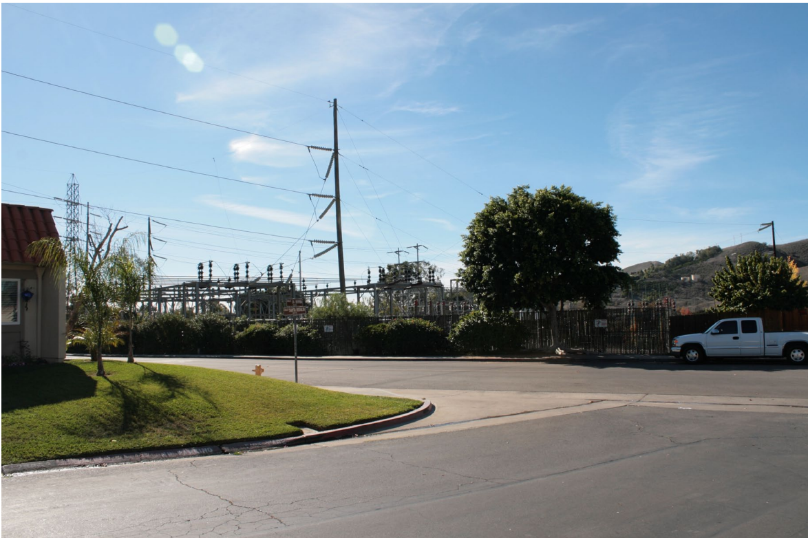
8. Calle la Bomba at Calle Santa Rosalia looking southwest
