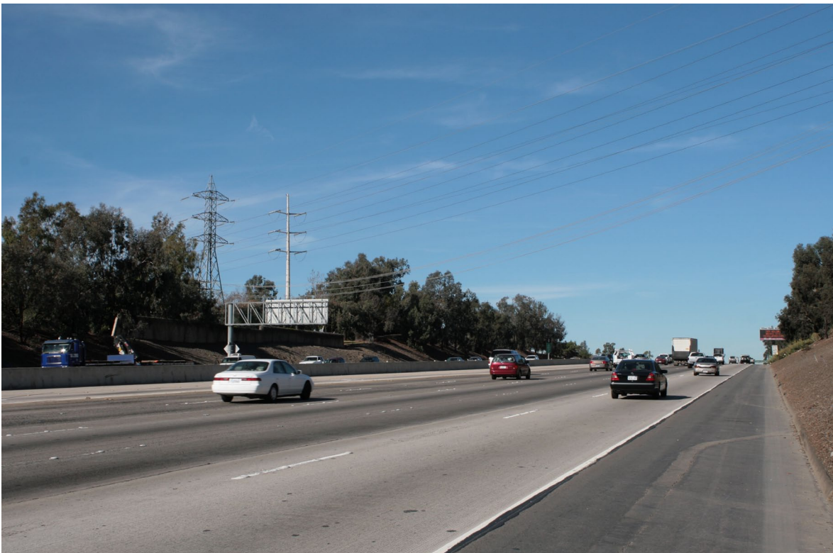
10. Interstate 5 northbound looking north
