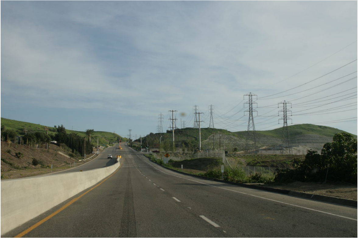
23. La Pata Avenue (east of San Juan Hills High School) looking south
