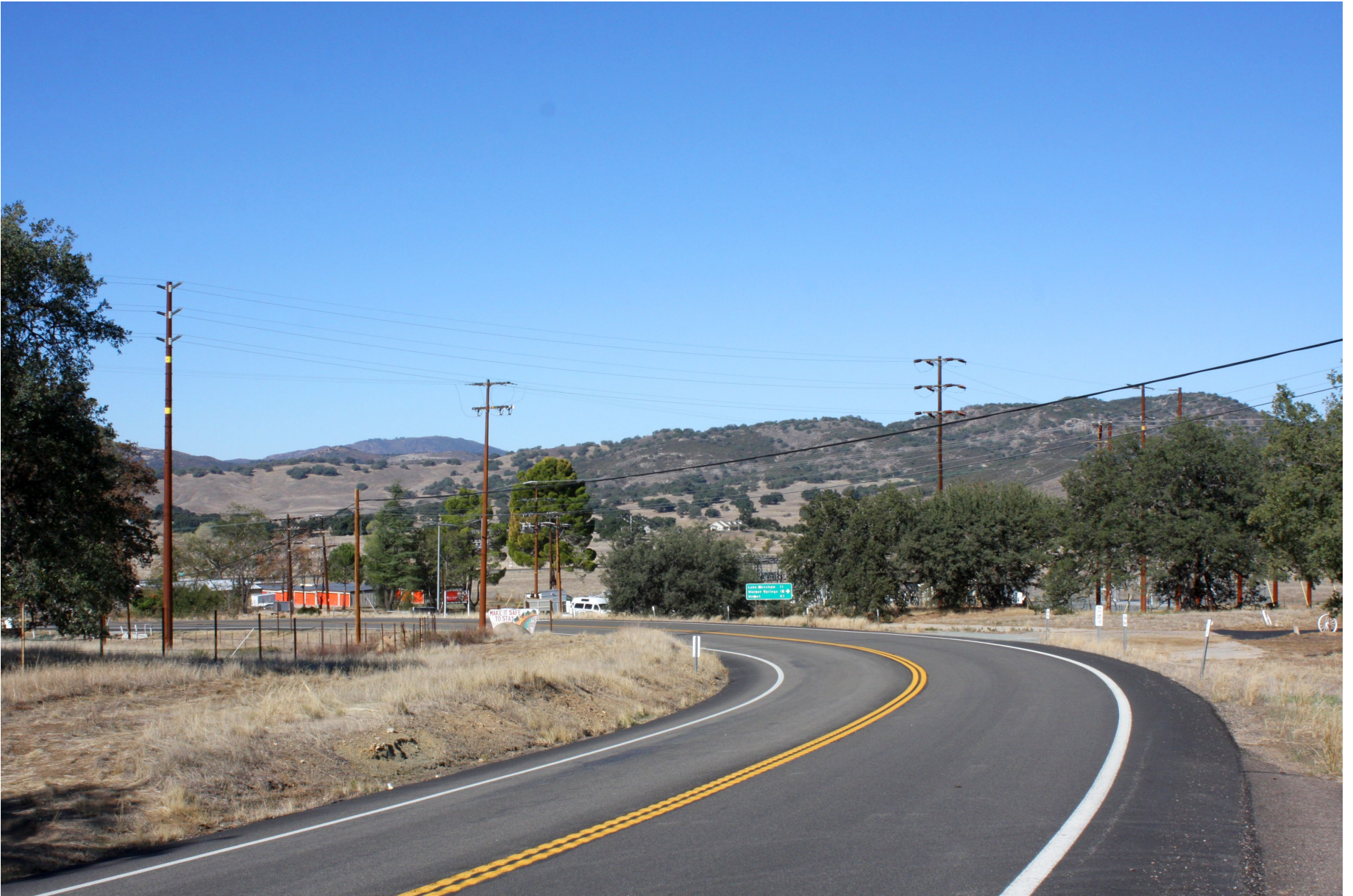
Existing View from Hwy 78/79 in Santa Ysabel looking northwest (VP 18)
