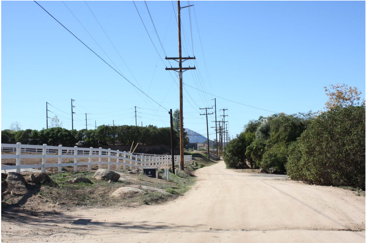
Photograph 1. Creelman Lane at Sixes Court looking west toward substation (Landscape Unit 1)
