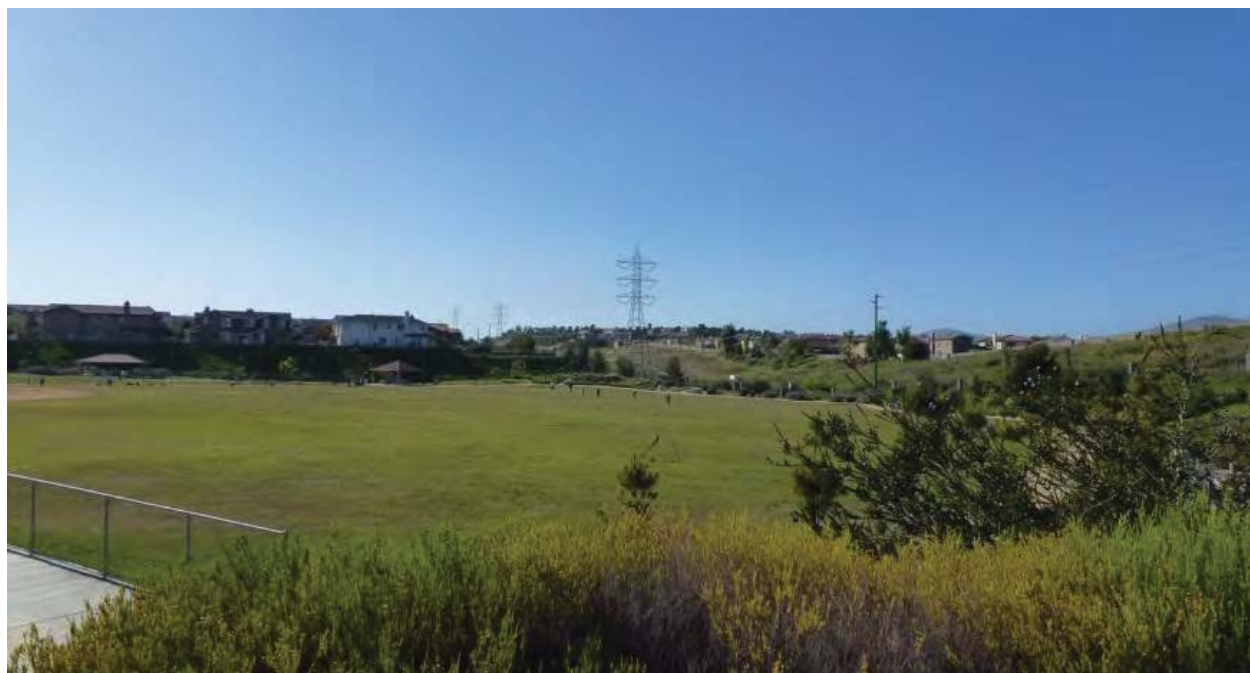
Figure 4.1-12: View North toward the Transmission Corridor
