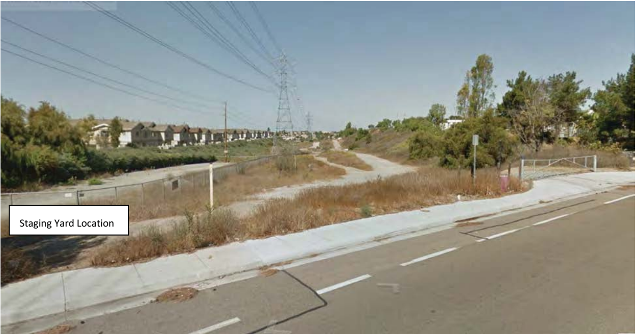
Figure 4.1-15: View of Eastlake Parkway Staging Yard from Eastlake Parkway
