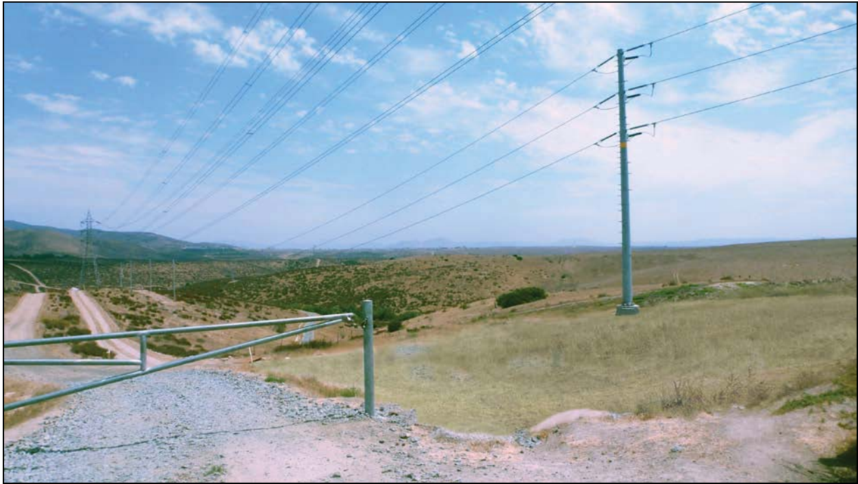
Figure 4.1-29: Key View 9: View Looking Southeast at Hunte Parkway/Transmission Corridor
