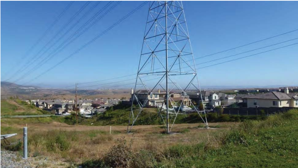
Figure 4.1-11: View South along the Transmission Corridor
