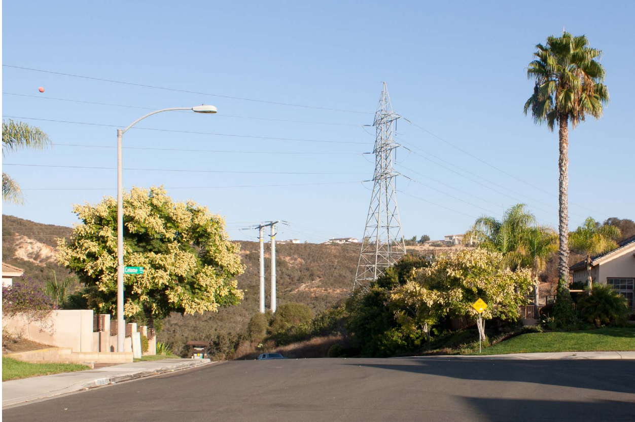
18. Park Village Road near Celome Way looking northwest (Segment C-D Junction) *
