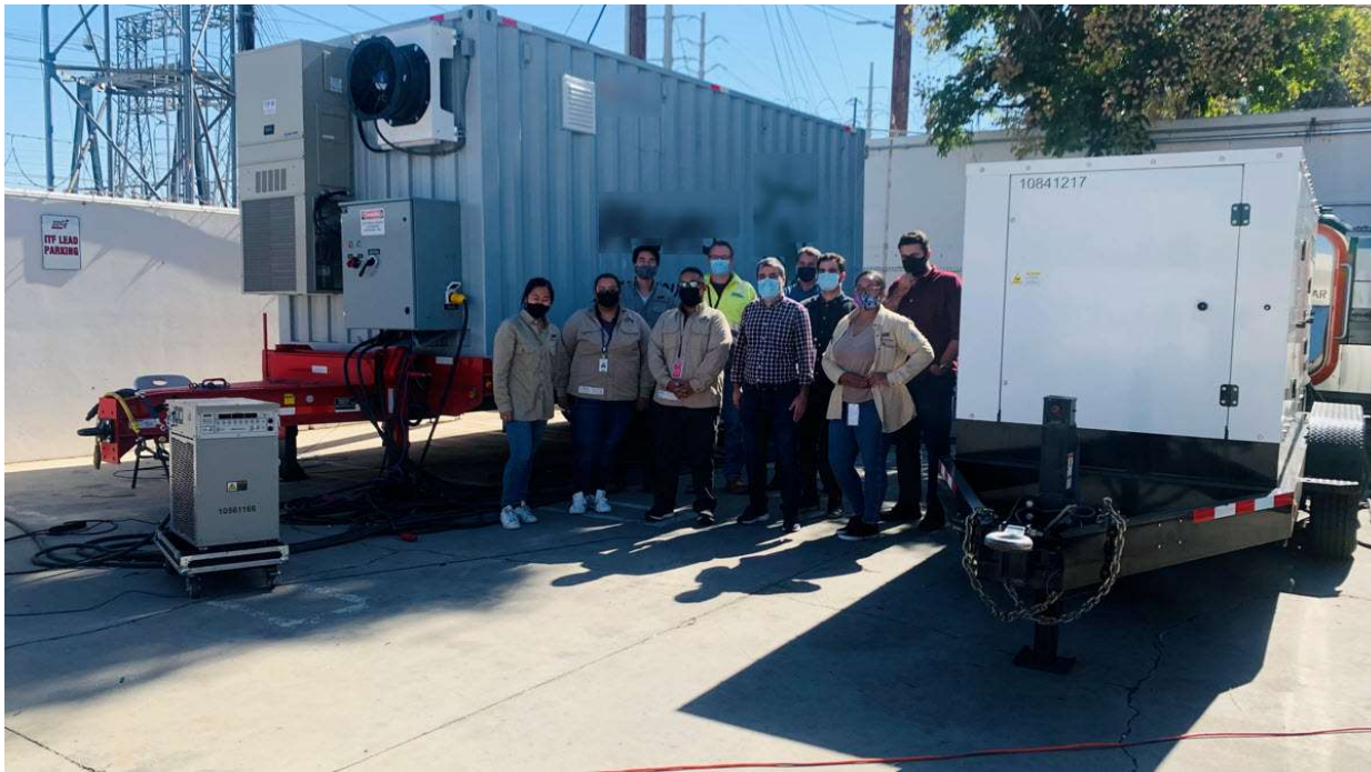
100 kW/525 kWh (only 1 string available)
