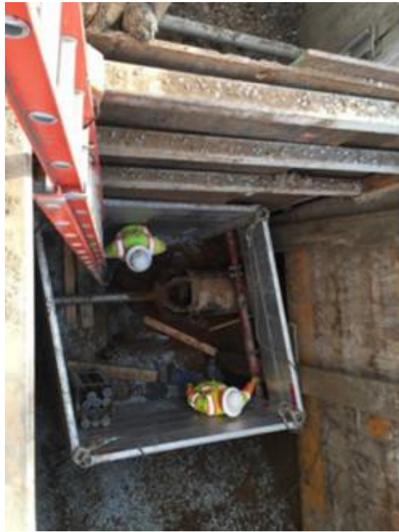
Figure 7: Jack and Bore Pit
