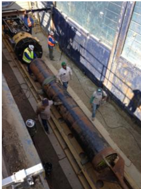
Figure 8: Jack and Bore Operation
