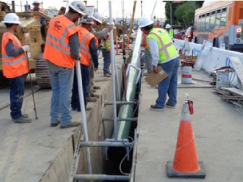
Figure 2: Lowering Pipe in Congested City Area
