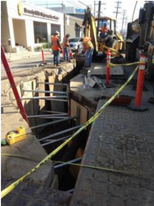
Figure 1: Trenching in Urban Location
