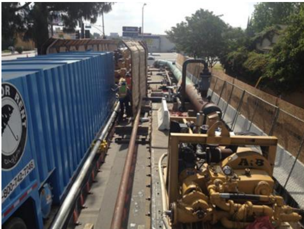
Figure 11: Hydrotest Set Up with Sound Proofing to Minimize Noise Complaints (located behind Baker tank)
