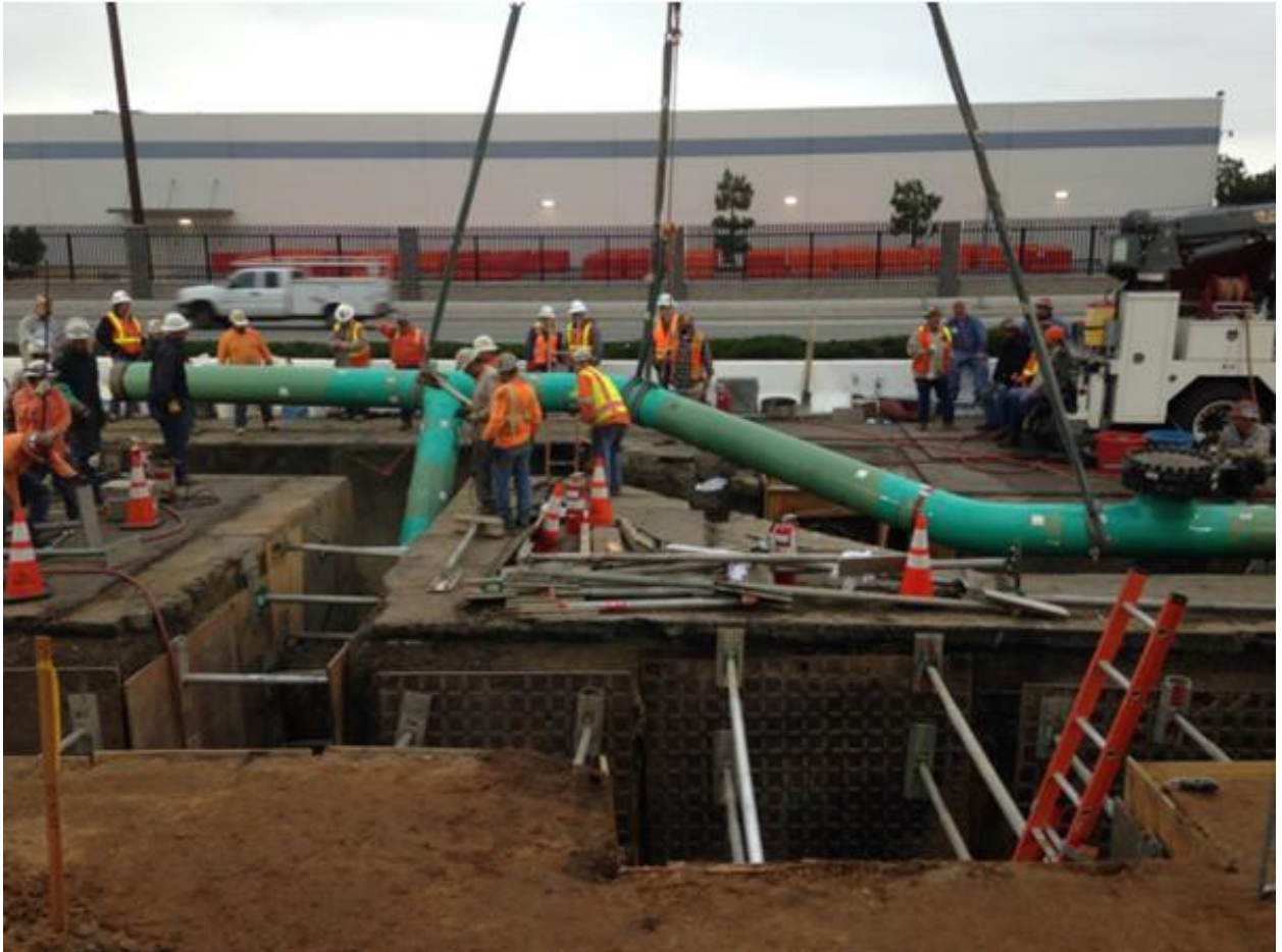
Figure 9: Lowering Section of Pipe into Trench
