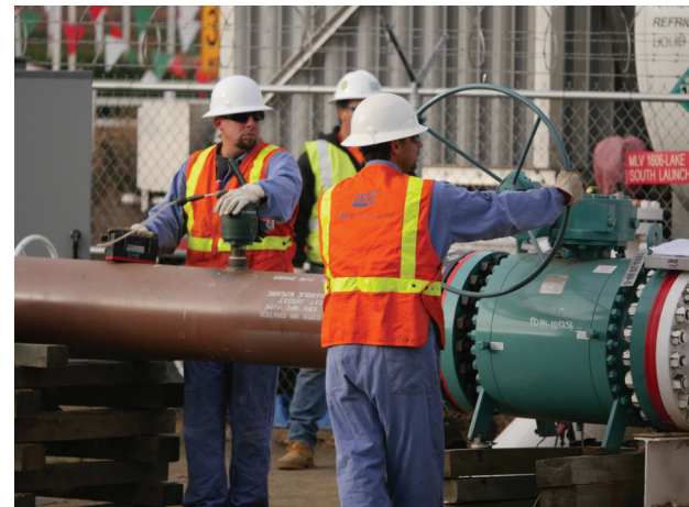
SDG&E has upgraded more than 23 miles of transmission pipeline in San Diego County as part of our Pipeline Safety Enhancement Plan.
