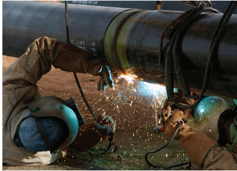
Workers carefully weld two pipeline sections together.
